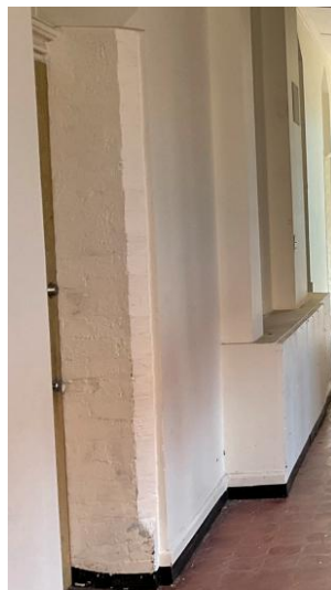
Ground floor north verandah
