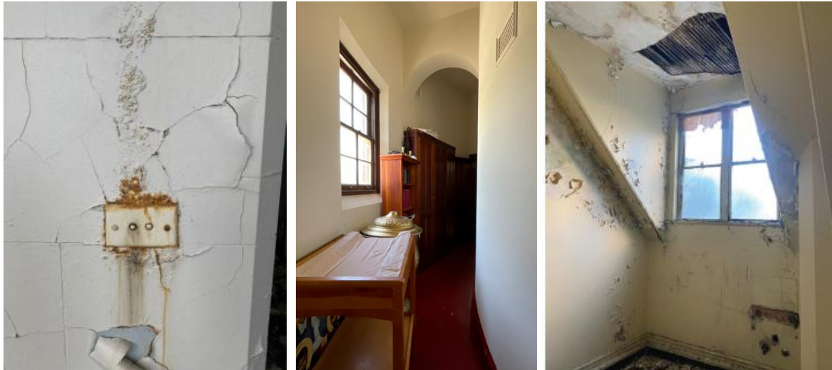
Ground floor, south verandah
