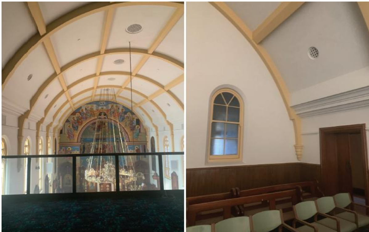
Figure 90 Looking east toward the apse from the balcony, showing the back wall of the balcony.
