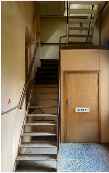
Figure 69 Various stair types Steel access stair, south wing
