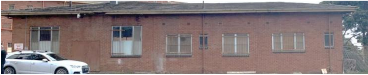
Figure 30 East Elevation of former child care building – a later addition to the laundry
