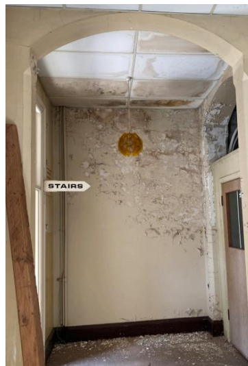
First floor north corridor
