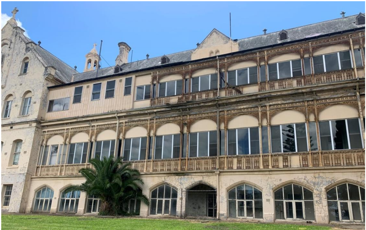
Figure 43 South link south side to berm
