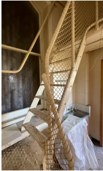
Steel stair to attic
