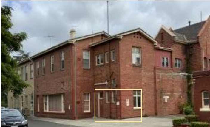
Figure 31 Additions at the north end of the south wing approximate location of 1907 bldg outlined in yellow
