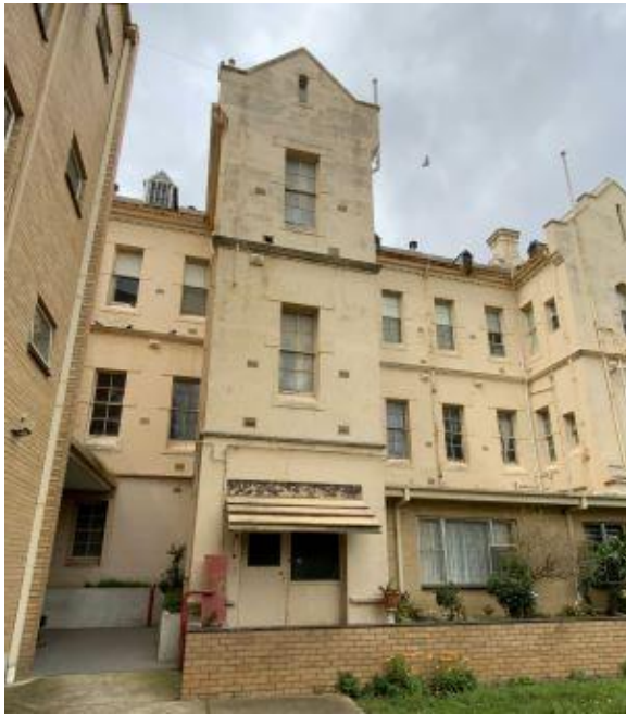
Figure 34 Demolish single-storey addition beside ablutions block and awning
