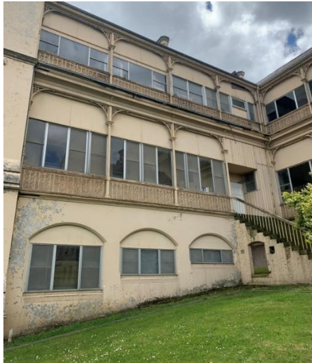
Figure 44 North wing verandah to berm
