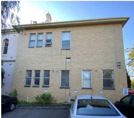
Figure 39 1960s addition at the end of the south wing
