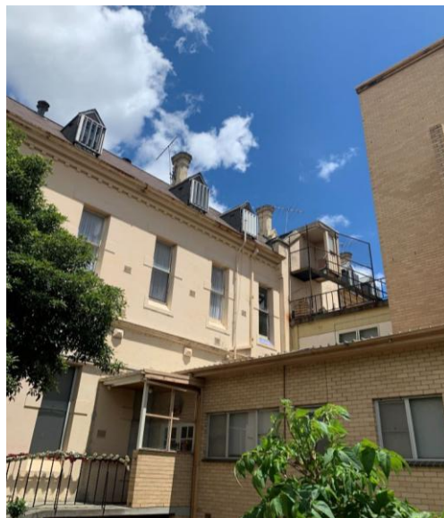
east side of connecting link
