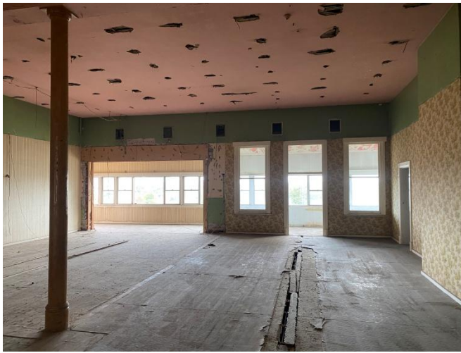
Figure 71 Existing condition of function room (1.103), wall to be removed on the right.
