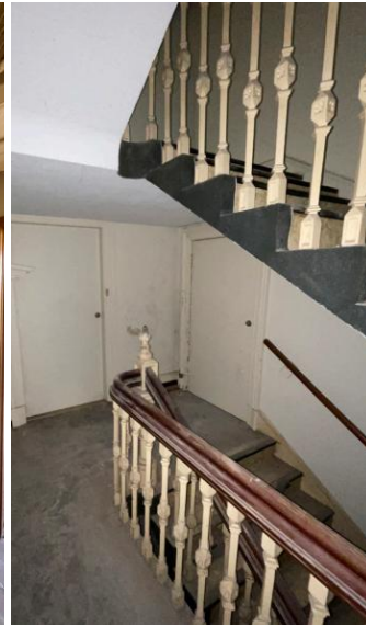
Stair 1, bluestone landing, vinyl and nosing over bluestone treads, ornate cast iron balusters
