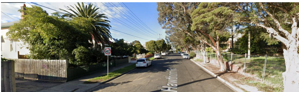
Figure 5 Looking up Hawthorn Road from St Georges Road, showing the former Little Sisters wall on the right. Image: Google Street View, 2019 (consistent with current conditions). Note the temporary fencing visible along the site boundary.
