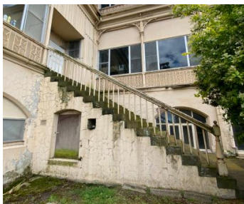
Figure 99: Central stair with bluestone treads and square cast-iron balusters
