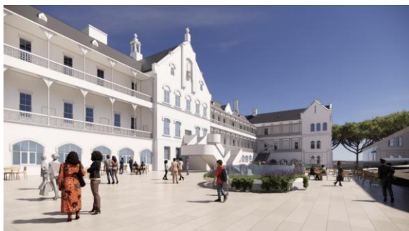
Figure 17 October 2023 presentation – hard-paved flat platía with glass pavilion illustrating loss of significant heritage features.
