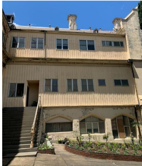
Figure 45 South wing verandah to berm
