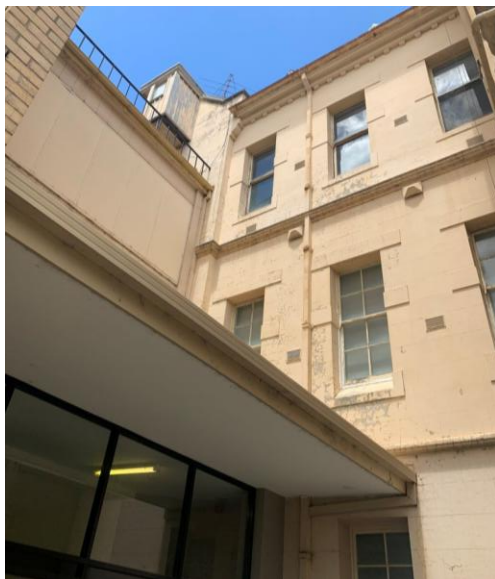
Figure 37 west side of connecting link
