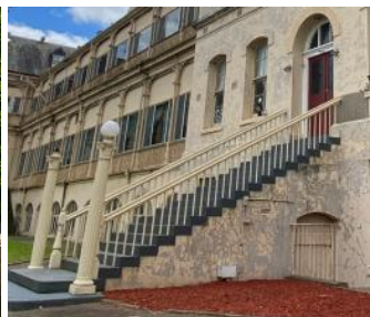
Figure 99: Central stair with bluestone treads and square cast-iron balusters
