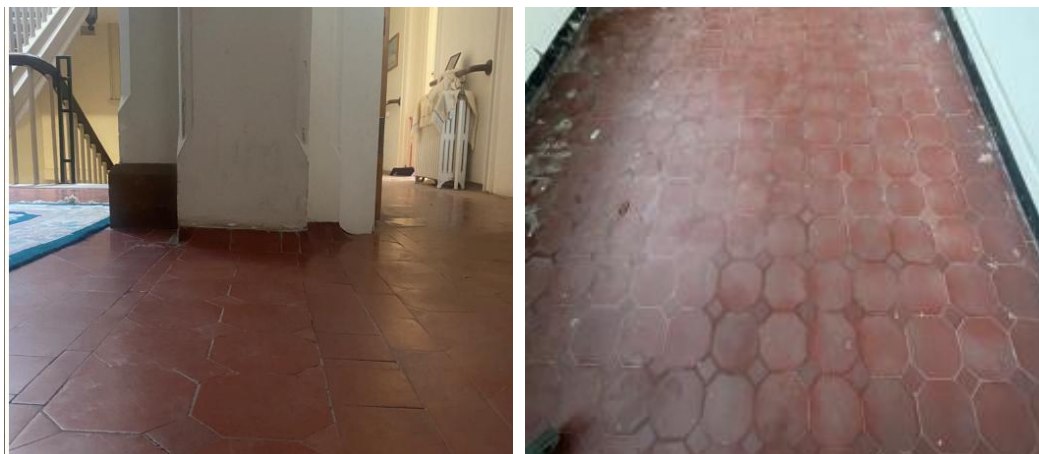
Room 1.114 – First floor, stage 2 and infill; Room G41.3 – Typical example.
