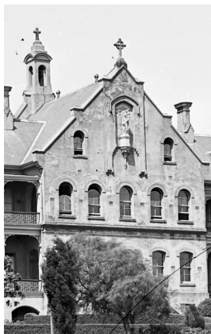
Façade of chapel in 1895-6
