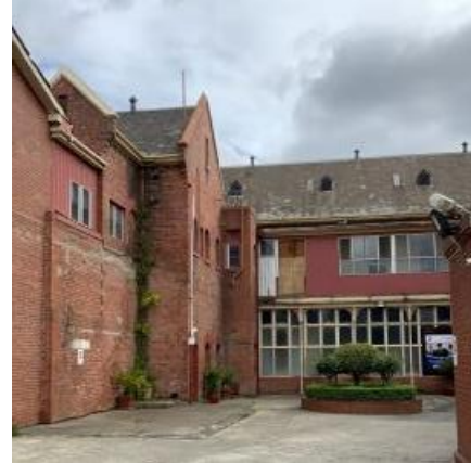
courtyard on the south side of the church
