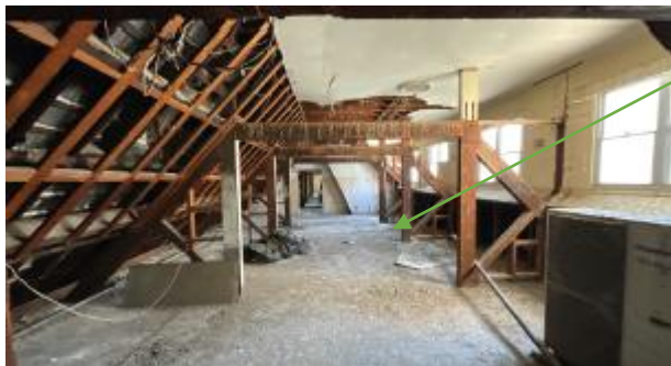
Figure 63 Section of modified wall on right to be partially removed.
