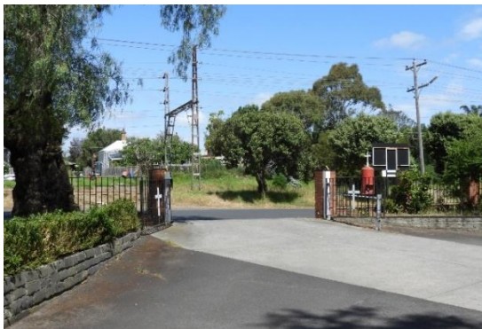
Gates and fence to Hartington St (NS)
