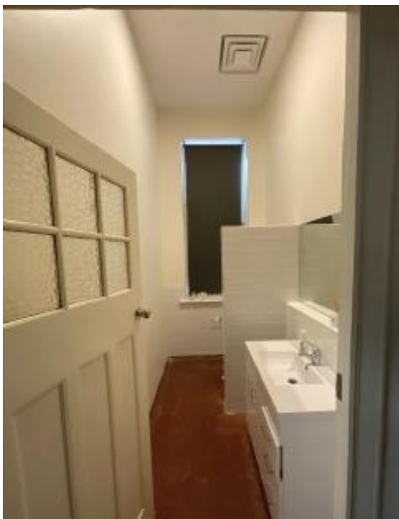
Figure 57 Corridor with bathroom infill
