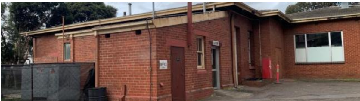
Figure 29 West elevation is currently used as a workshop and contains an early iron beam – no original roof forms
