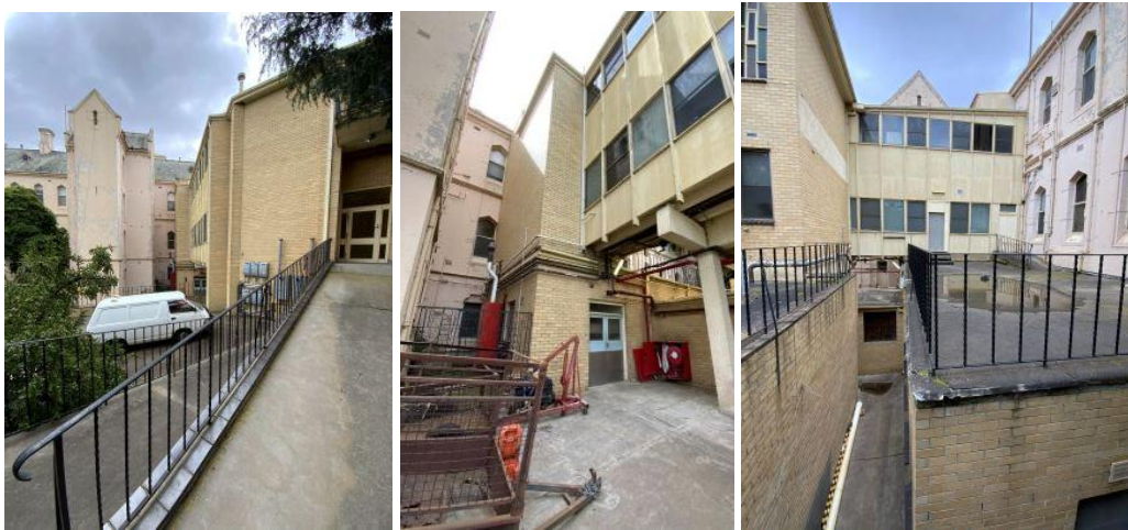
Figure 35 South side of new wing basement and link from south north side of new wing and link
