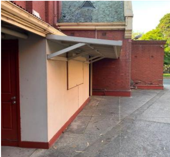
Figure 48 built-in section of verandah on east side of the church
