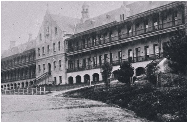
After completion of the third stage, loggia still open
