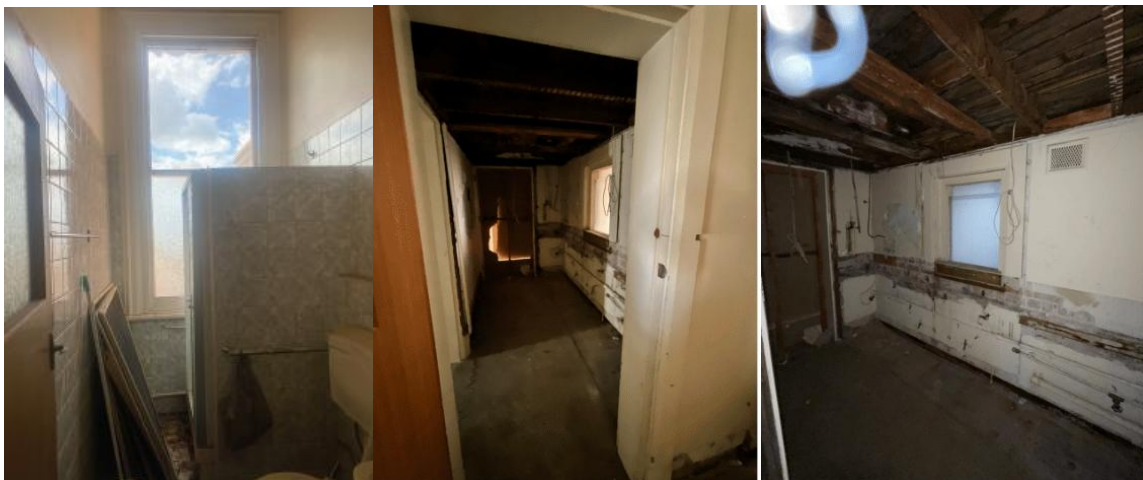
Figure 74. Bathroom installed in the corridor space
