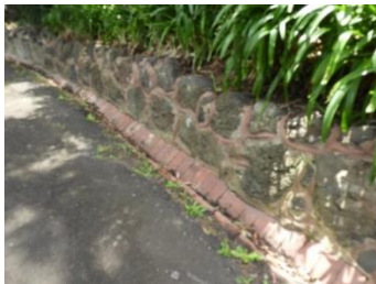
Brick drains (S)
