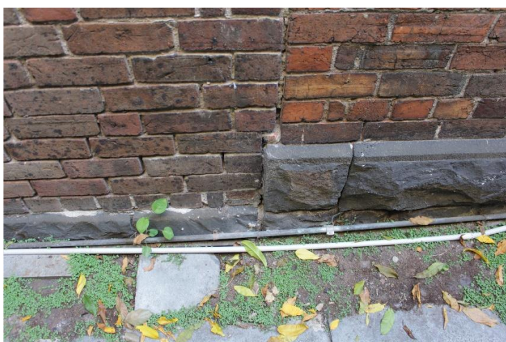
Figure 16 East elevation of rear wing showing the different basalt plinths and brickwork to 1869 (right) and circa 1880s (left) sections
