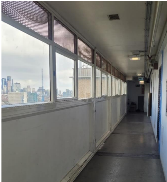
The original balcony access to the flats has been infilled with metal framing and glazing
