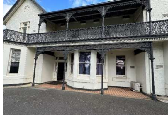
Figure 12 Lacework verandah to the north elevation. Note bay windows to ground level. Source: Trethowan Architecture, 2024.
