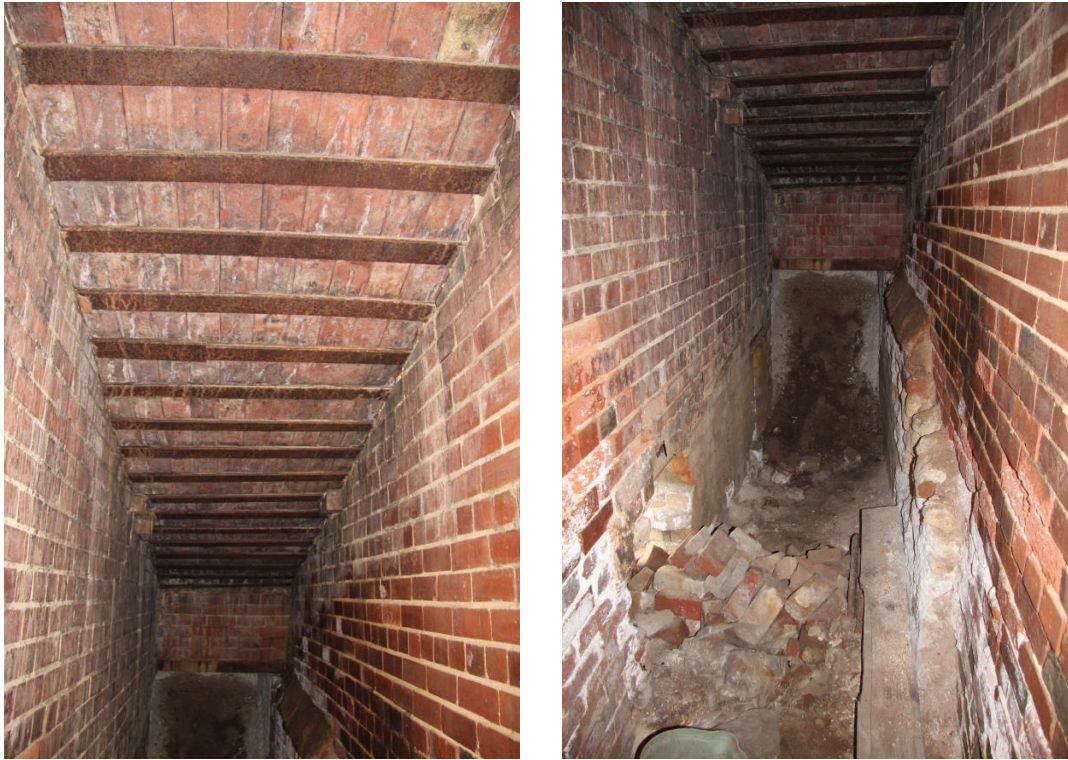
Figure 17 Interior of the fire tunnel remains Source: Lovell Chen archives, 2015
