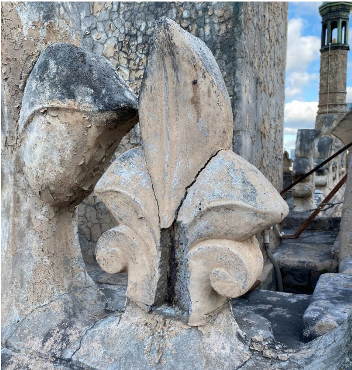
Figure 5 Spalling and cracker crenelations on the tower parapet.
