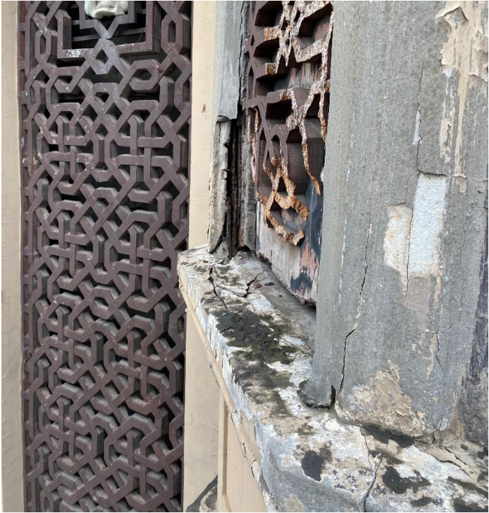
Figure 7 Canted bay columns busting apart as a result of corrosion of reinforcing.
