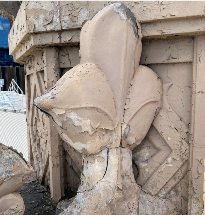
Figure 4 Parapet crenelations in poor condition and cracked through in a number of locations.
