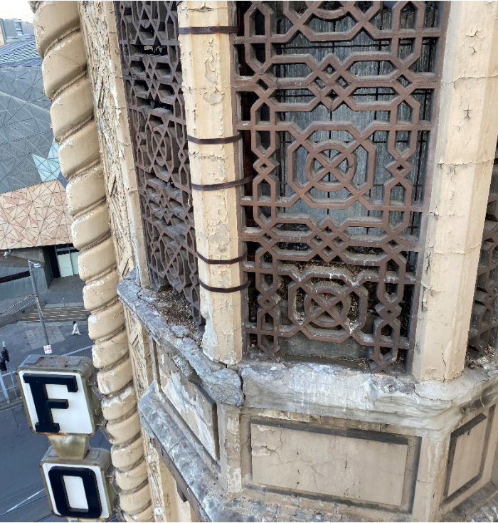
Figure 6 Dilapidated canted bay structure. Columns are vertically split due to corrosion of reinforcing and sills are spalling.
