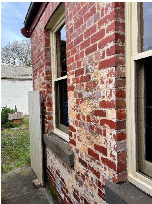
Figure 6: North elevation of the historic Cottage looking towards the Laneway.
