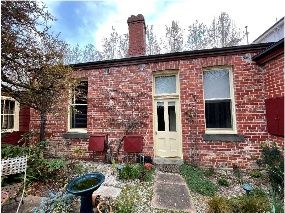
Figure 8: North elevation of amenities outbuilding.
