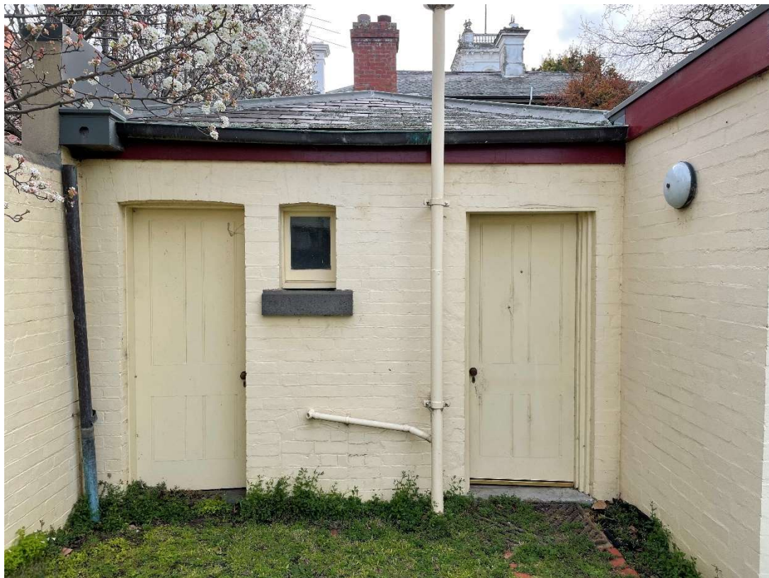
Figure 7: East elevation of amenities outbuilding viewed from Laneway.
