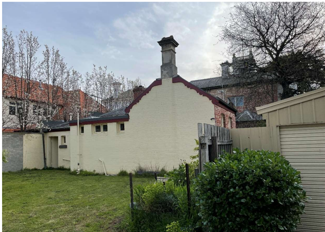
Figure 3: View from Laneway showing amenities outbuilding to left, the historic Cottage outbuilding with pitched roof and chimney to the right, and its contemporary addition in the centre.
