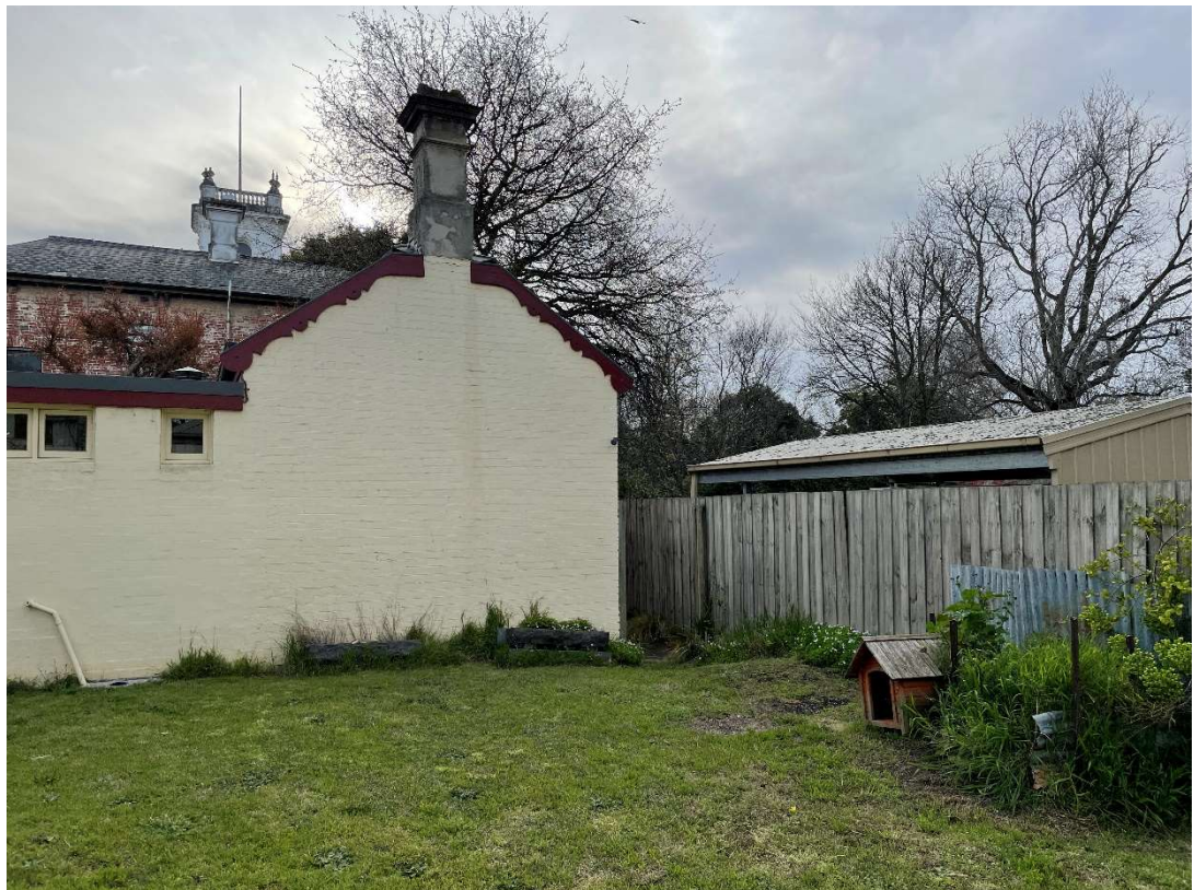
Figure 4: East elevation of the historic Cottage viewed from the Laneway. Contemporary addition on the left.
