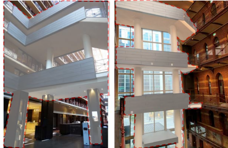
Existing bridges and structure to be removed.
