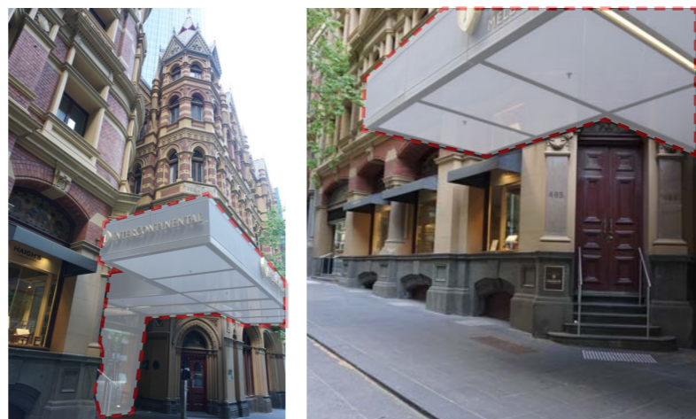
Removal of Collins St Canopy and airlock
