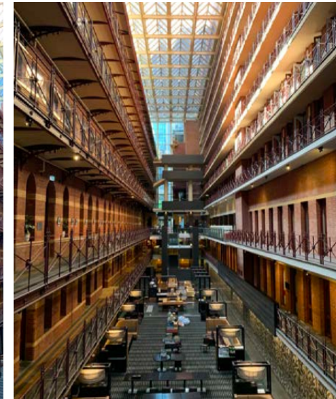
Raised timber floor structure at base of atrium currently serving as a hotel dining space
