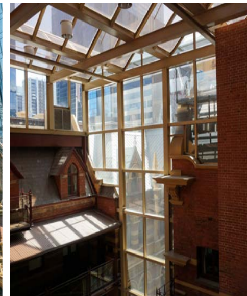
Top of glass atrium, Collins Street façade
