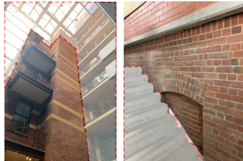
1980's addition and fire stairs removed from Winfield Building rear
