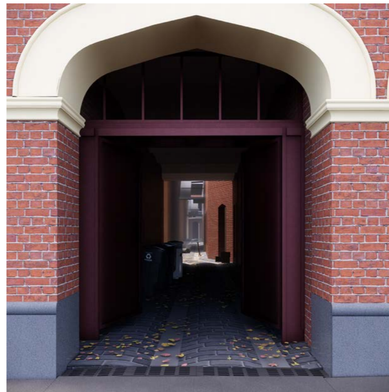
Existing Service Laneway
