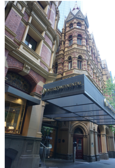
Collins Street Entry. Winfield to the left and Rialto to the right.
