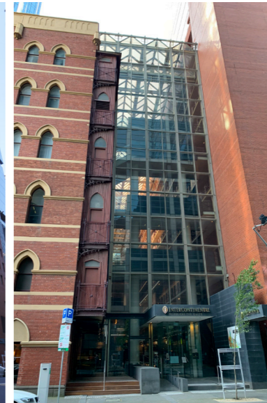
High Rise Urinals on the Eastern Wall of the Rialto and the 1980's glass atrium in the centre of photo.
