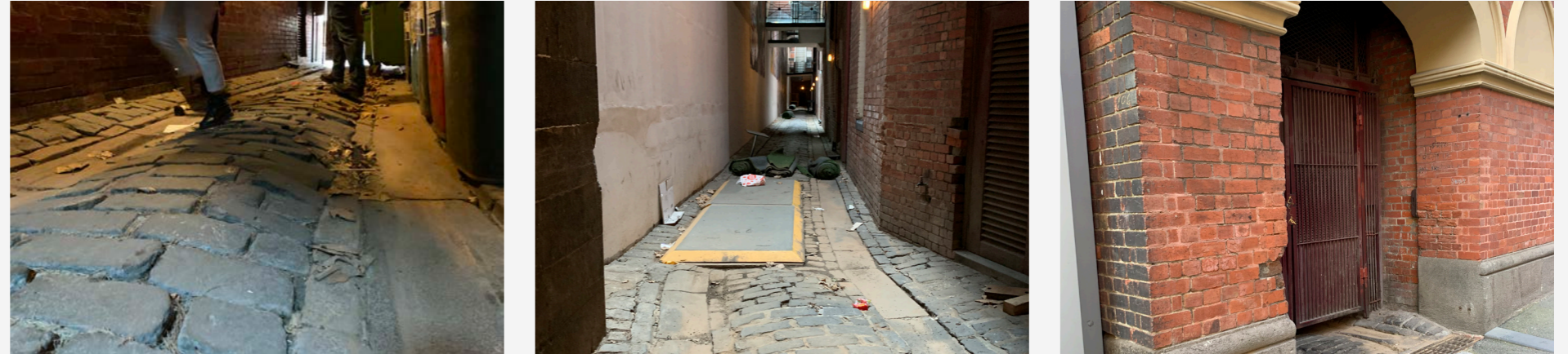
Existing Condition Photos
