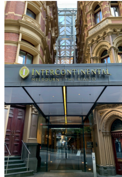
Collins Street Entry. Winfield to the left and Rialto to the right
