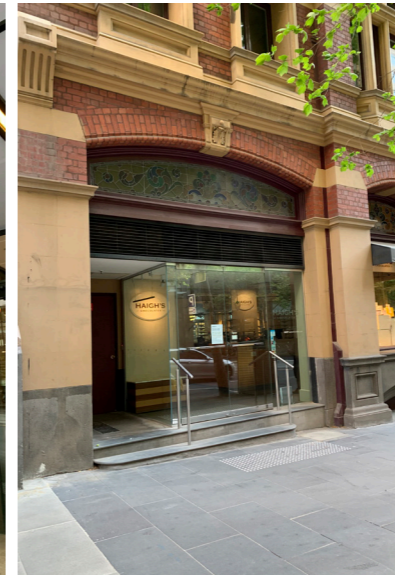
Modified entry to Winfield on the East border of the site on Collins
