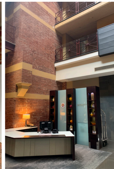
Southern wall of the Winfield adjacent to the 80s addition
