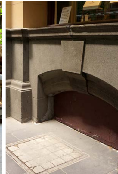
Old bluestone lightwell into basement of the Winfield
