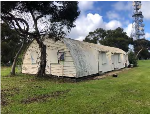
Figure 5: External of Nissen Hut. All openings have been boarded up with plywood. All windows and doors have previously been replaced with aluminium
