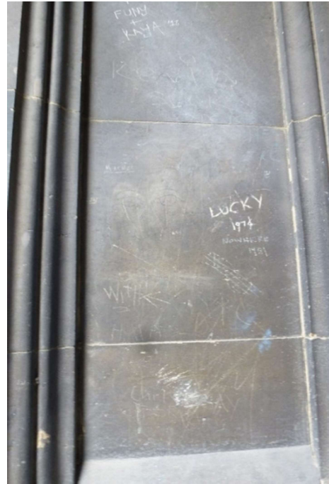
This stone has been damaged by graffiti which has been scratched through a layer of soot and patina. Sanding is not an acceptable treatment for this type of damage because it will remove and roughen the finely finished surface and damage the adjoining mouldings. A conservator or conservation stonemason will be able to clean the wall which will disguise the graffiti.
