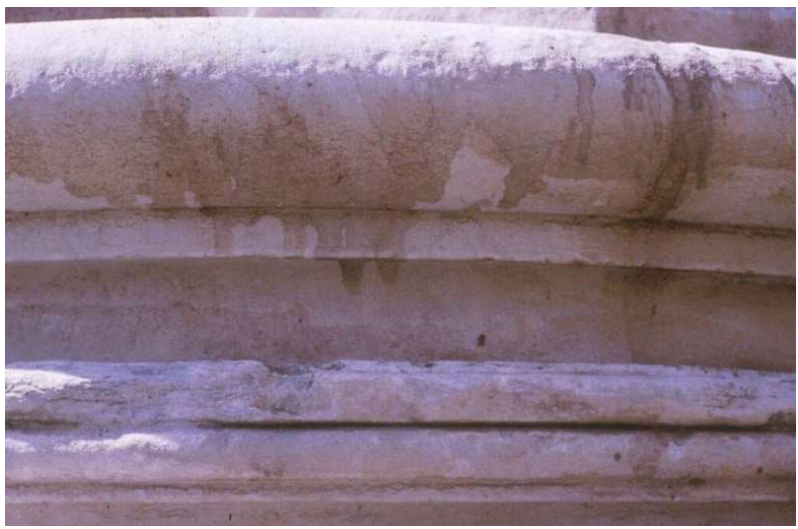
Badly applied or unsuitable graffiti barriers have darkened and discoloured these stones
