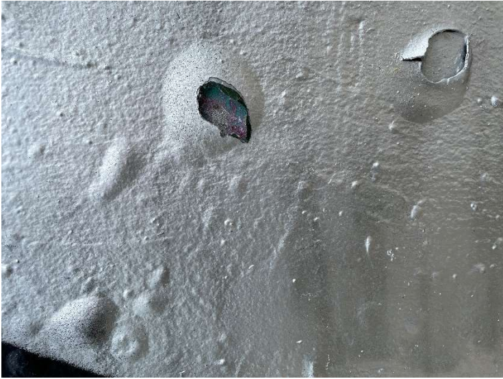
Repeated painting over graffiti, will quickly lead to the build-up of heavy layers of paint. This will peel, flake or bubble due to incompatibility between the graffiti layers and the wall paint.
