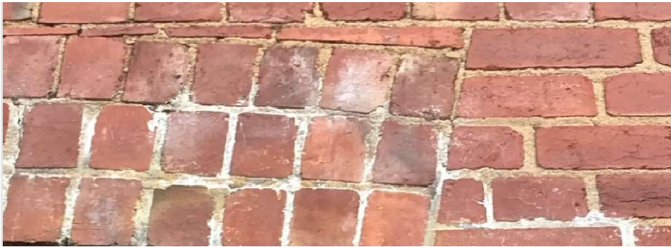
Residues of paint stripper that was not fully rinsed off.
