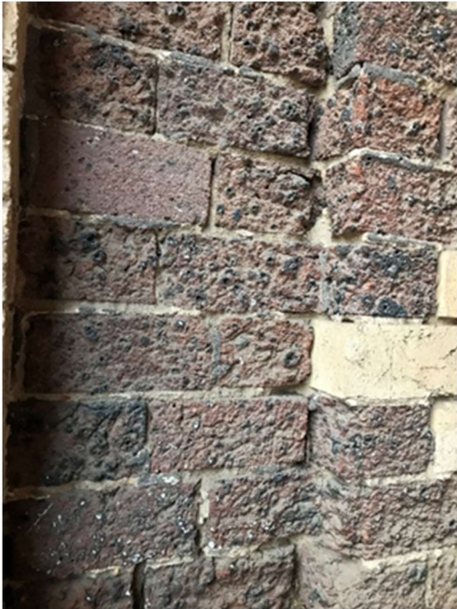
Bricks which have been severely damaged by pressure blasting. The 'fire skin' or hard exterior has been removed from the brick. This will lead to water entering the building causing damp or mould.
