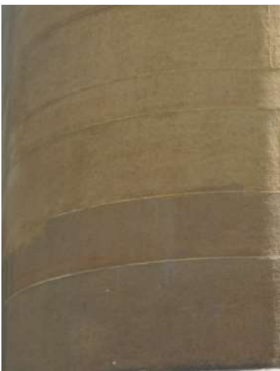
Badly applied or unsuitable graffiti barriers have darkened and discoloured these stones
