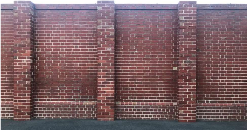
This wall is suffering from rising damp, visible as darker areas. This has been caused by repointing with a non-breathable mortar.
