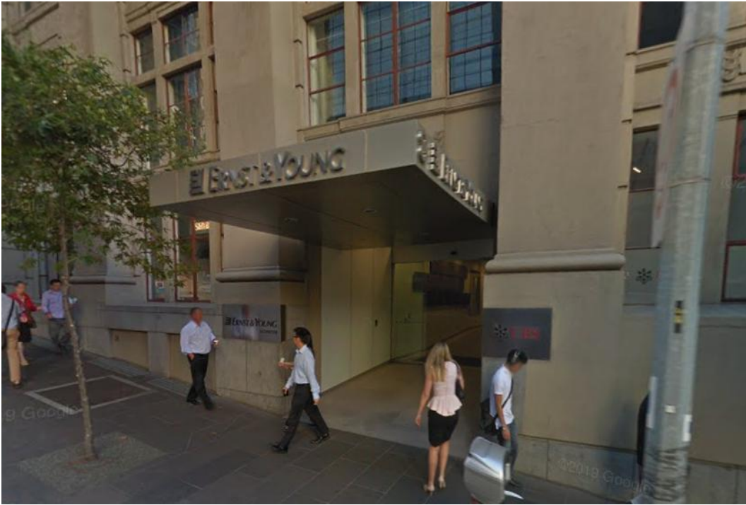
Figure 5 Image of the canopy which had been in place since at least 2007, showing the lighting and soffit Source: Google Street view, March 2013
