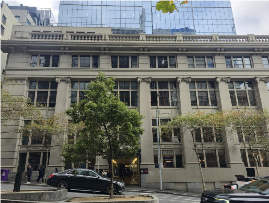
Figure 7 View from the opposite side of Exhibition Street showing the current arrangement of the Exhibition Street entry and canopy Source: Lovell Chen, July 2026
