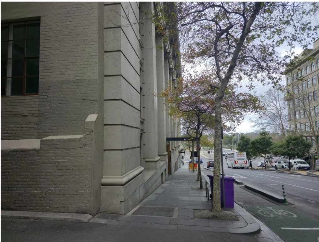
Figure 9 View of the existing canopy looking south along Exhibition Street from Sargood Lane Source: Lovell Chen, July 2026
