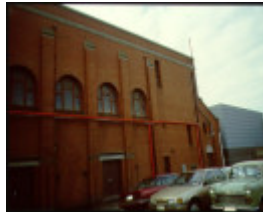
H01967 cathedral hall south elevation
