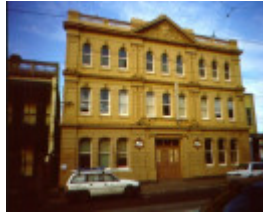
H01967 1cathedral hall facade
