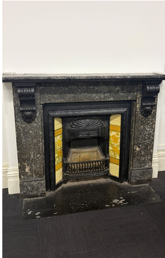
Figure 9 – Fireplace to the east wall of Room G.10.
