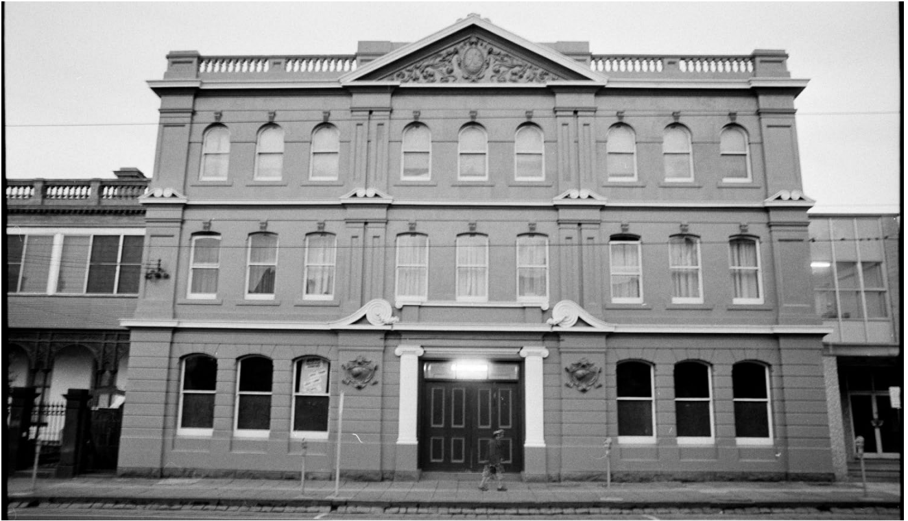
Figure 17 – Cathedral Hall in c.1970.
