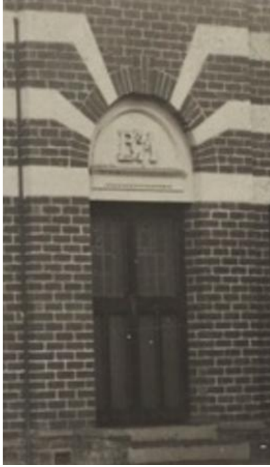
Figure 51 (Left): extract from photograph showing external door to Lobby2. Source: Exterior View Showing Courtyard Behind Church Street Facade, 1920-6, SLV, H92.401/9)
