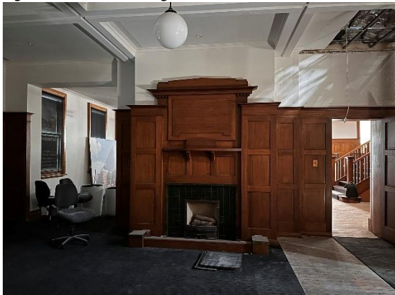
Figure 64: Rm 11 looking south.
