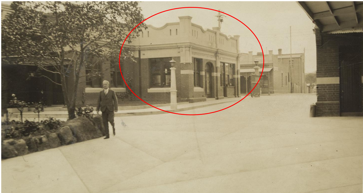
Figure 18: Image of the entrance and south side of the office buildings, showing further changes to this façade. The south façade appears to have been extended further across the site entrance (circled red). Source: Inside Grounds of Bryant & May Factory, Richmond, Nov 1928, SLV, H92.401/433.
