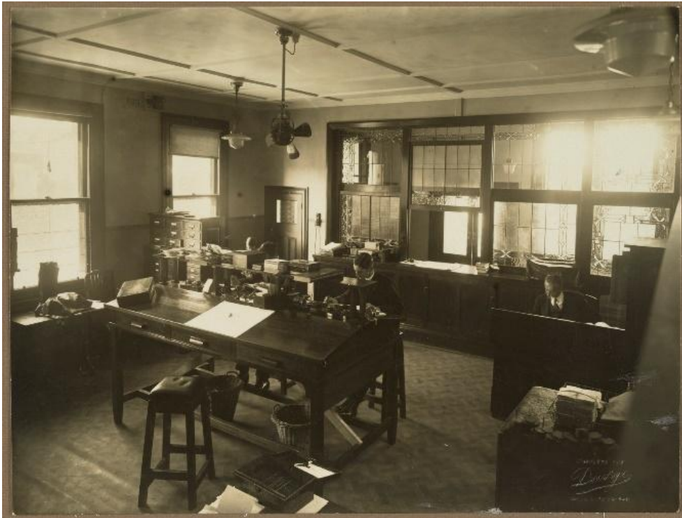
Figure 54: Image of the office area taken 1920s likely looking southeast towards the early entrance lobby. (Source: Men at Work in Office Area of Factory, Probably Bryant & May, c1927, SLV, H92.401/343)
