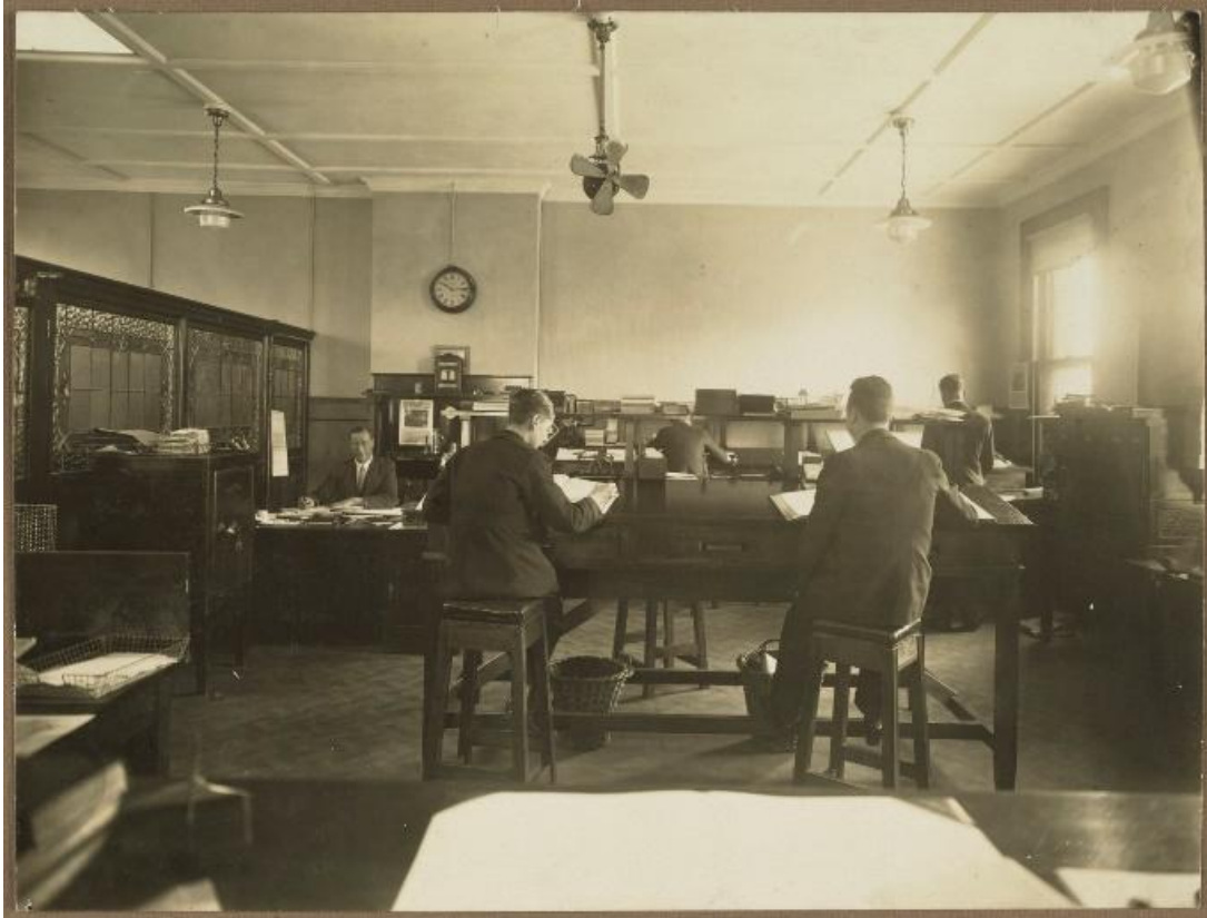
Figure 20: Image of an office area at Bryant & May, likely taken c.1927 looking north in Room 10 as shown on application drawings. Source: Men at Work in Office Area of Factory, Probably Bryant & May, c1927, SLV, H92.401/342.
