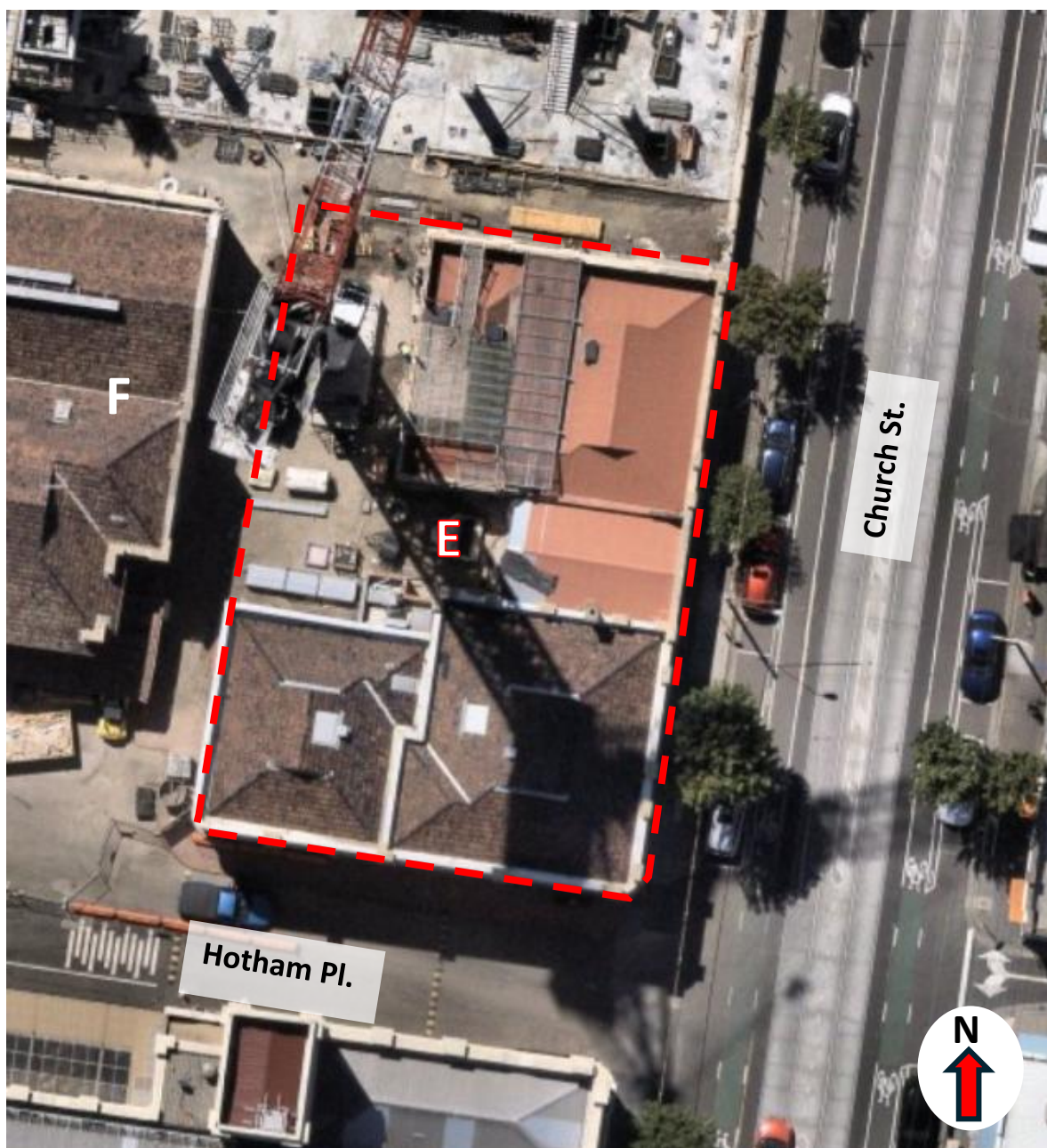
Figure 2: Aerial image of the former Administration Building (subject site) taken on 14 February 2026. Source: NearMap 2026.
