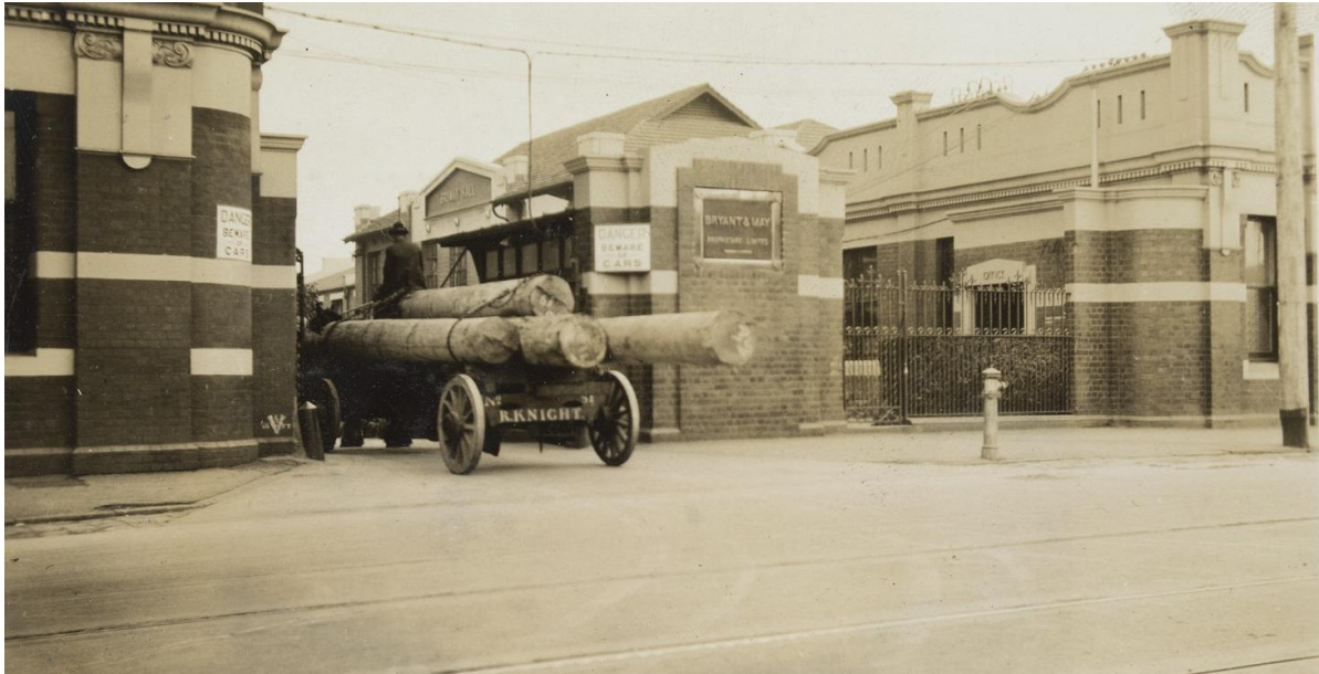
Figure 17: Image of the entrance to Church Street, showing portions of the south and east elevation of the Administration Building after the façade was extended along the former dining room. Source: Two Horses Pulling Wagon Load Of Logs into Bryant & May Richmond Picture, 1920s, SLV, H92.401/421.
