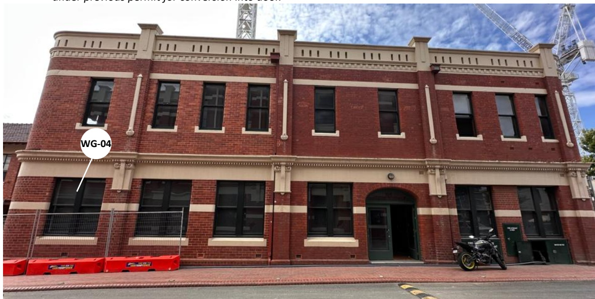
Figure 90: Subject site as seen from the south showing affected window.
