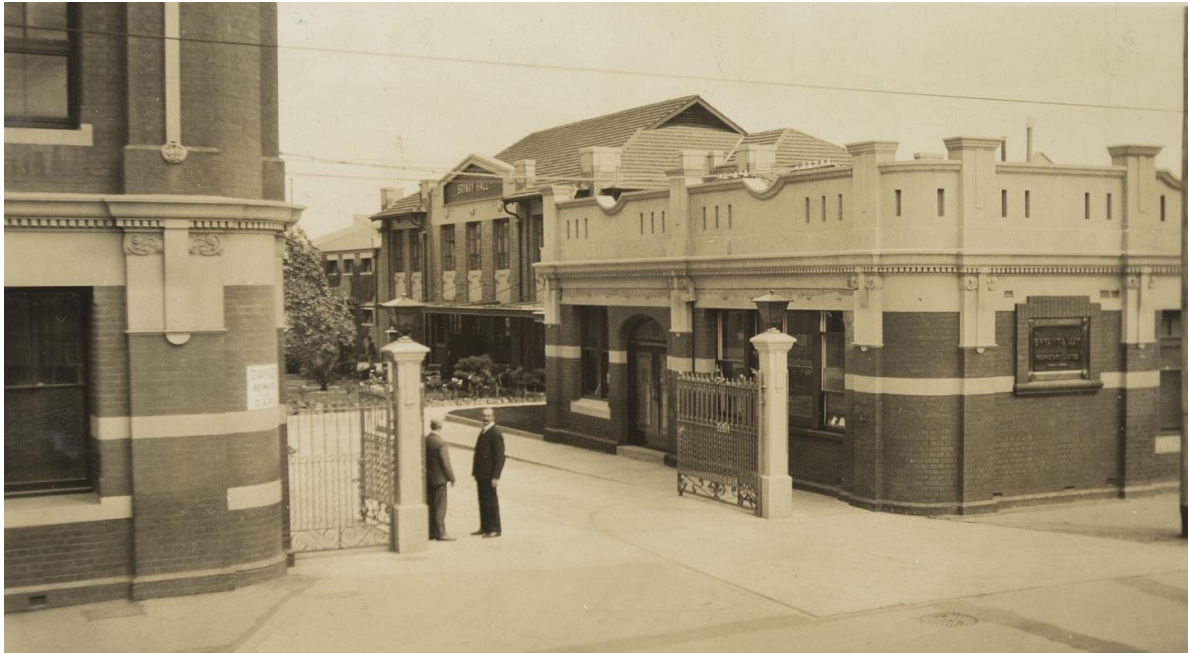
Figure 19: Image showing portions of the south and east facades of the offices (pictured right of image), with the south façade further extended and changes shown to the east façade, including the relocation of the plaque. Source: Looking Through Gates at Bryant & May, Richmond, to Brymay Hall, 1928 , SLV, H92.401/435.
