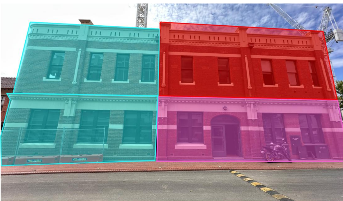
Figure 37: Phases of development at the former Administration Building - Eastern (Church Street) elevation. Source: Google Streetview with RRCD overlays.
