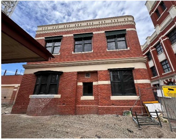
Figure 44: Western elevation of Administration Building.
