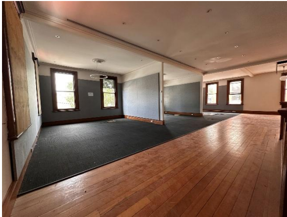
Figure 73: Stair landing level 1 looking south-east.
