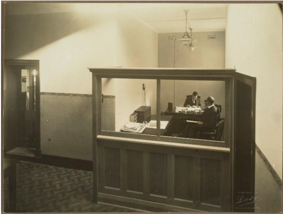
Figure 27: Image of an office area at Bryant & May, likely taken c.1935 on level 1 looking west from room 17 on the application documents, prior to the c.1942-1950 extension. Source: Office Area of Factory, Probably Bryant & May, 1920-30, SLV, Algernon Darge, H92.401/344.
