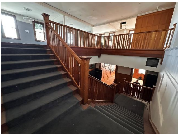
Figure 71: Stair landing looking south-east.
