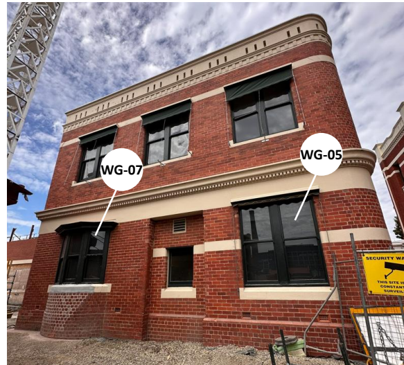
Figure 89: Subject site as seen from the west showing affected windows.
