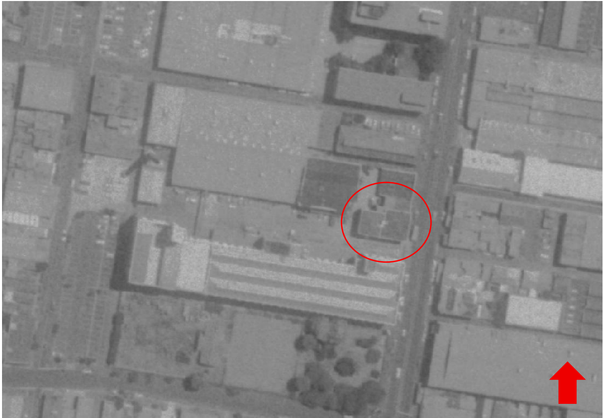
Figure 25: January 1983 aerial of the Bryant & May Match Factory, with the Administration Building circled red. Note that the ground floor and the first floor have been extended to the western portion (originally the dining room). Source: Run Unknown, Frame 791, Geoscience.
