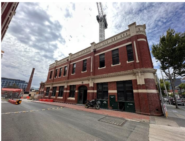
Figure 42: Southern elevation of Administration Building as seen from the southeast in Hotham Place.
