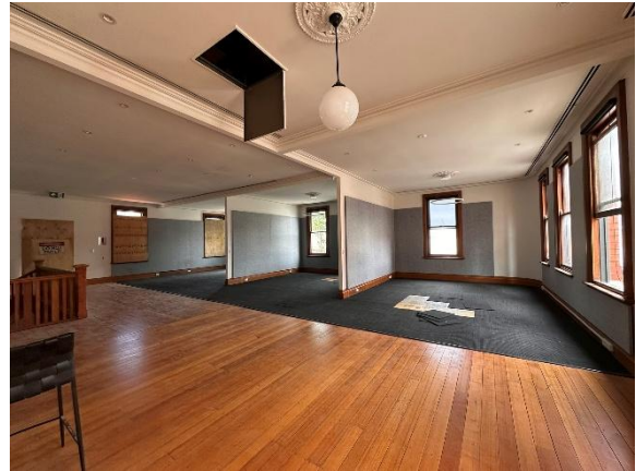
Figure 74: Corridor rm 17 looking east.
