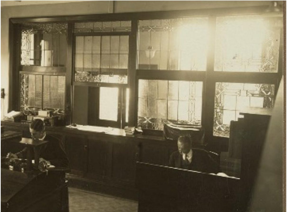
Figure 53: Extract from image of the office area showing partition at entrance lobby c.1927. (Source: Men at Work in Office Area of Factory, Probably Bryant & May, c1927, SLV, H92.401/343)
