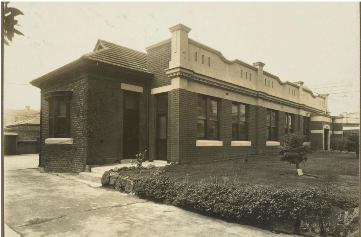
Figure 16: Administration Building after southern façade was extended further south. Source: Building and Garden at Factory, Possibly Bryant & May, c1910-32, SLV, H92.401/339.
