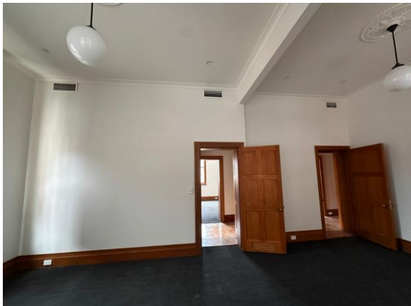
Figure 83: Room 3 - c.1942-1950 office addition - looking north.
