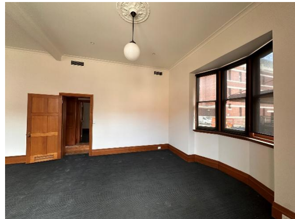
Figure 69: Rm 05 looking southwest.
