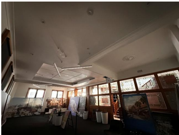
Figure 62: Rm 10 looking southwest.
