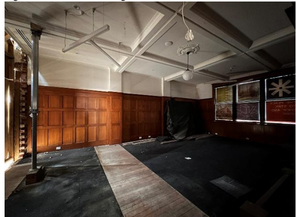
Figure 65: Rm 11 looking northeast.
