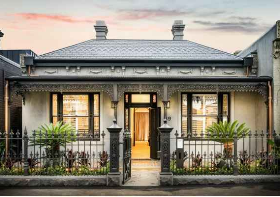
9a James Hardie 'Easylap' fibre cement sheet cladding and fascia in Dulux 'Natural White Half' (a) 'Monument' (b)
