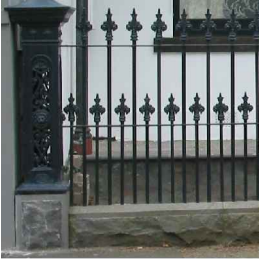
4 Existing cast iron elements, window frames & front door in Dulux Super Enamel semi-gloss 'Monument - C29'
