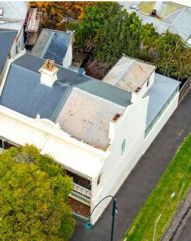
existing rusted iron roof sheeting with chimney features removed
