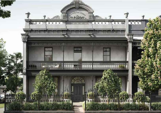
7 New powder coated aluminium window frames in Dulux 'Monument' with enviro double glazing
