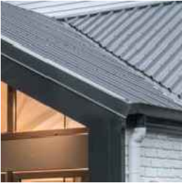
10 Lysaght klip-lok steel roofing and fascia in Colorbond 'Monument'
