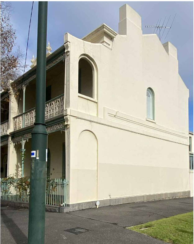
existing front facade with two-tone paint, cracks in render, exposed conduits and street light pole
