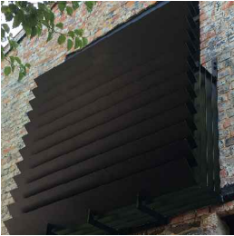
8 Aluminium louvered screening - Colorbond 'Monument'
