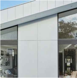
9a James Hardie 'Easylap' fibre cement sheet cladding and fascia in Dulux 'Natural White Half' (a) 'Monument' (b)
