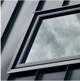
7 New powder coated aluminium window frames in Dulux 'Monument' with enviro double glazing
