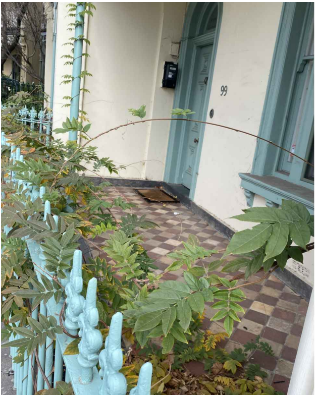
existing verandah tiles with excessive grout and cracked front facade (tiles likely been relayed poorly)
