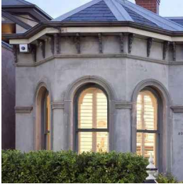
1 Investigate existing paint finishes on existing form. Remove paint and reinstate original render. Make good
