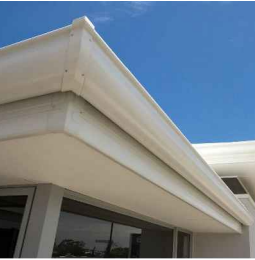
11 New gutters and downpipes in Colorbond 'Surfmist'
