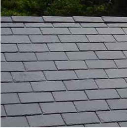
2 Reinstate slate tiles with Glendyne slate roof tiles. COS colour to match neighbouring no.97
