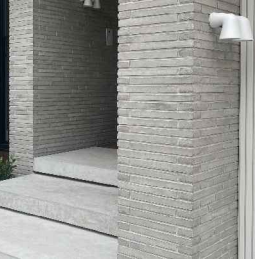
5 AHBP '011 (LB) S' Blended Bricks 400mm L x 40mm H x 90mm D
