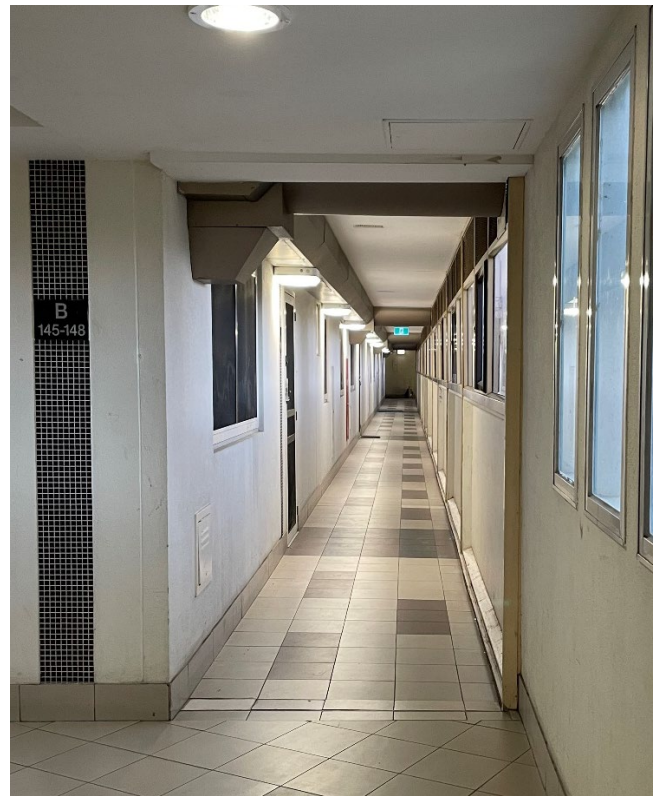
Corridor B, Level 12. Original balcony access to flats infilled with metal and glazing to form corridor
