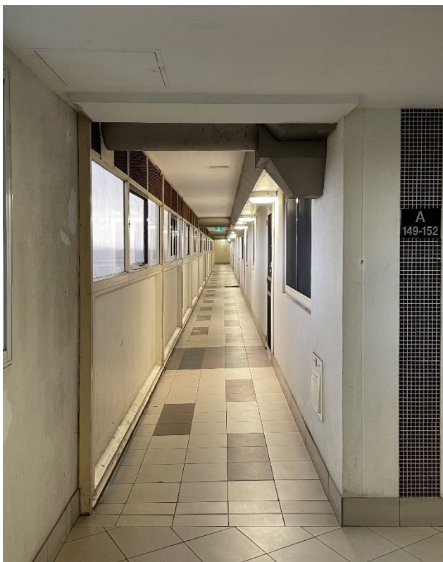
Corridor A, Level 12. Original balcony access to flats infilled with metal and glazing to form corridor
