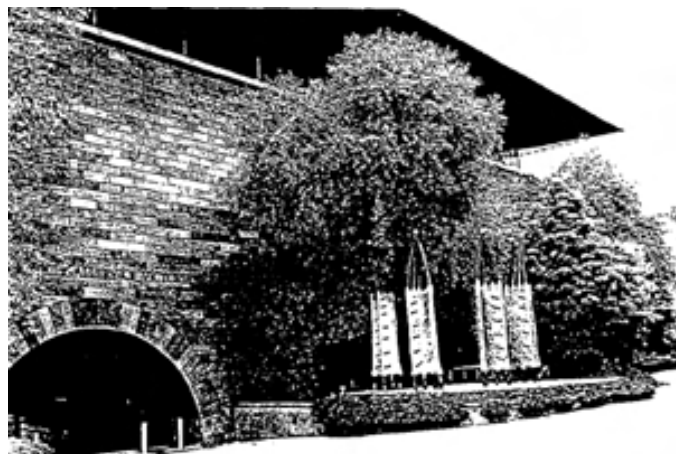
Fig 28: North West view, 1997. Note the raised planter in lieu of the moat here and the sloping ground towards the "mousehole" to accommodate the raised level for the State Theatre (Figure 90, NGV CMP Meredith Gould Architects, 1998).
