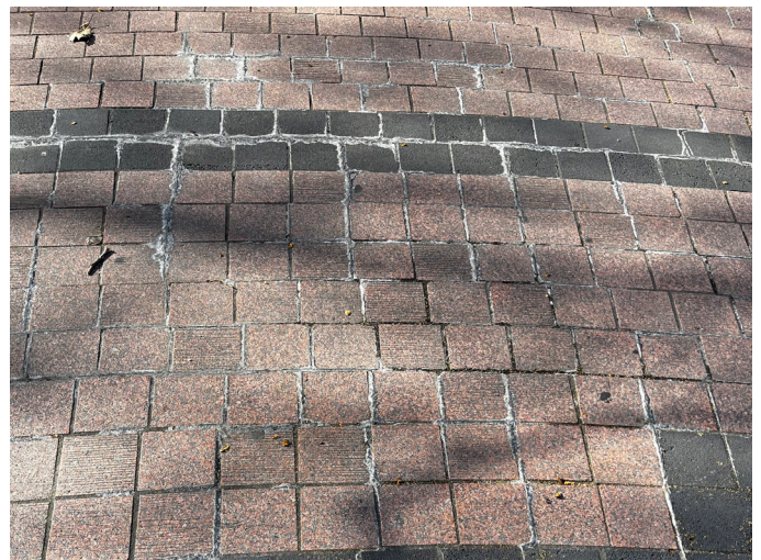
Fig 15: Detail view of localised paver and grout repair to Theatres Building forecourt (Hassell, 2024).
