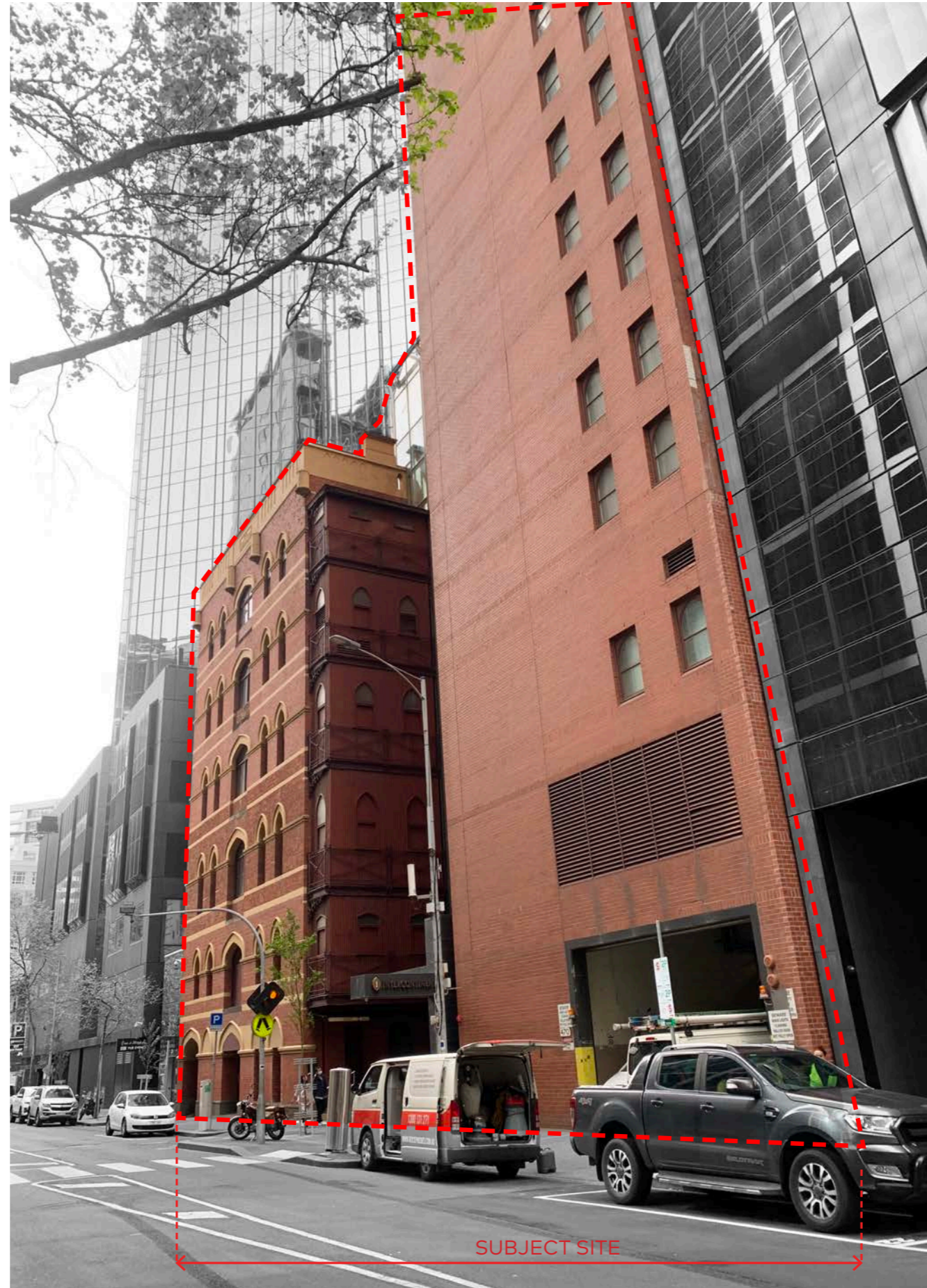
View 2 - Flinders Lane Frontages. The Heritage Rialto frontage (Left), 1980's addition (Right)
