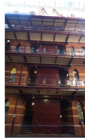
WATER POWERED LIFTS
