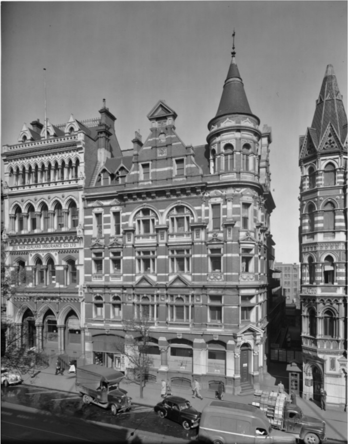
The Winfield Building, 1954. Source: State Library of Victoria.
