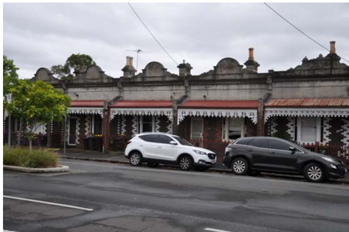
second chimney of 114 is not visible from Paterson Street (view from across street, title line of northern properties, looking south-west)
