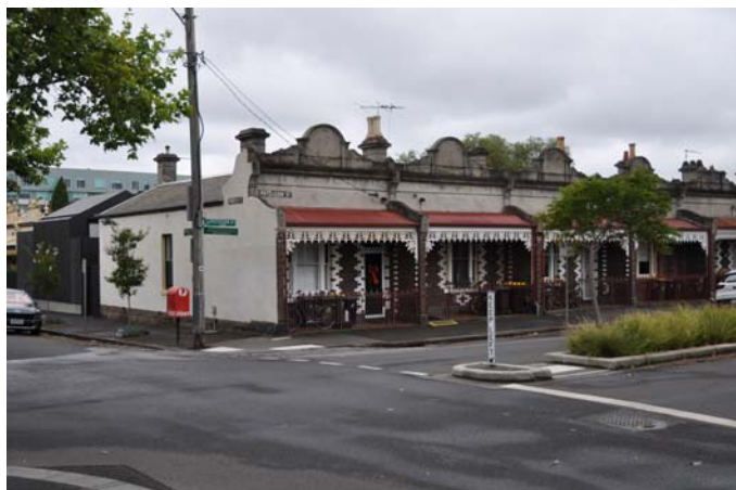
second chimney of 114 is not visible from Paterson Street (view from across street, title line of northern properties, looking south-east)
