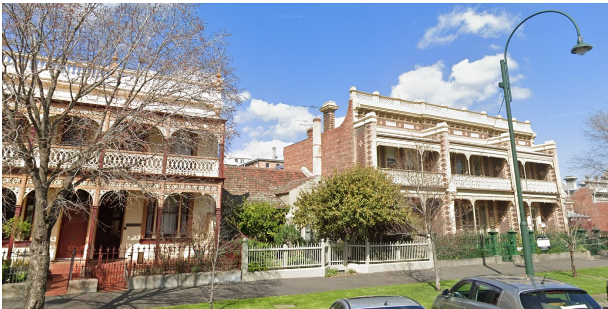
Figure 4 View of east wall of 61 St Vincents Pl above the roof of No. 59 next door looking to the rear of the Biltmore behind (Google Streetview)
