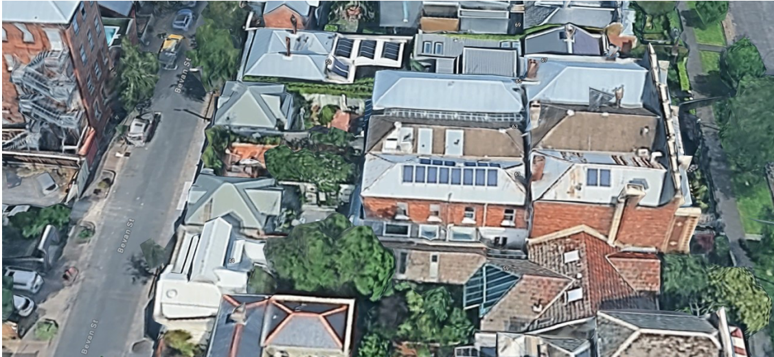
Figure 5 Aerial view of 61 St Vincents Pl and roof of No. 59 next door (Google)
