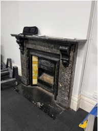
H. MARBLE FIREPLACE WITH DECORATIVE MOULDED MANTEL, TILE FLOOR. OVERALL 1200MM H x 1800MM L
