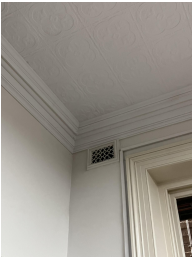
G. PAINTED TIMBER MOULDED CORNICE WITH STEPPED AND COVED SECTIONS. DECORATIVE PRESSED METAL CEILING PANELS.
