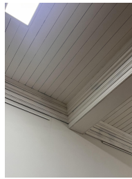
D. PAINTED TIMBER MOULDED CORNICE WITH STEPPED AND COVERED SECTIONS. PAINTED TIMBER TONGUE & GROOVE BOARD CEILING.
