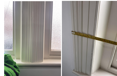
F. PAINTED TIMBER DOUBLE HUNG WINDOWS. TIMBER MOULDED ARCHITRAVE FRAME. TIMBER PROJECTING WINDOW STOOL WITH NOSE PROFILE. OBSCURE PATTERNED GLAZING.
