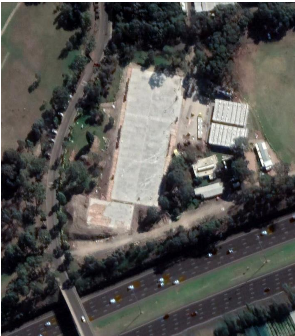
Figure 12: March 2022 satellite imagery of the central section of the impact zone showing the continuing construction of the Yarra Bend Park – Fairlea Reserve – Netball Courts.
