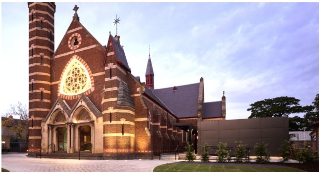
Former St Georges Uniting Church, converted into a performing arts centre with a modern/dark metal clad toilets and change rooms visible to the right.
