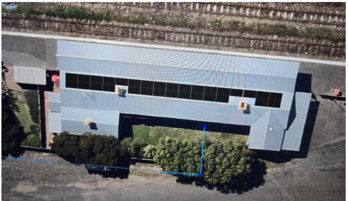
Photo 3. Aerial view of the station with 31 solar panels installed. The blue line is the route of the underground power supply cable from the meter board, located to the west of the station building to the station building.
