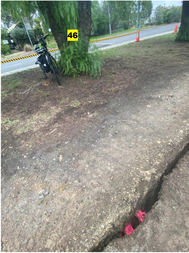
Image 11: Tree 46, 2 roots located 80mm, 100mm
