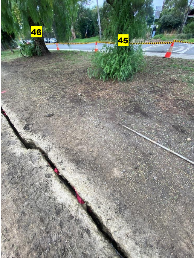
Image 10: Tree 45, 2 roots located 60mm, 80mm.
