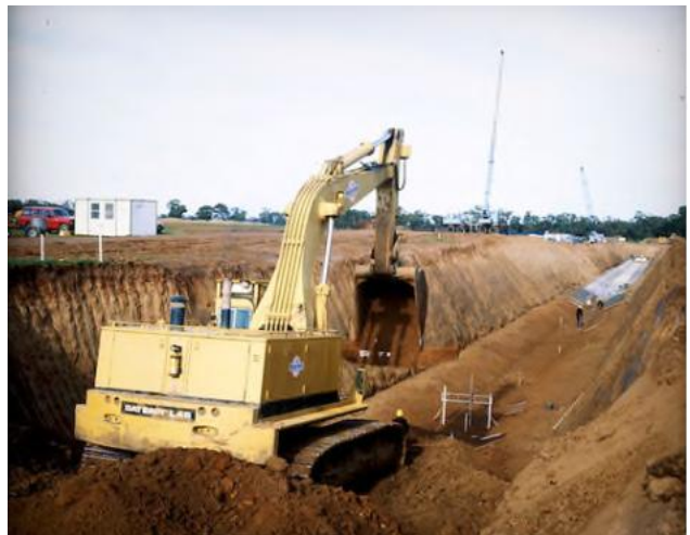
Figure 2-10: Construction of the WTS at Farm Road on 25 July 1983 (Melbourne Water)
