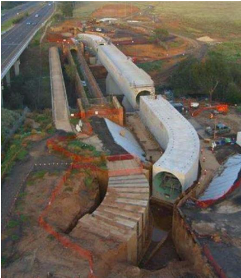
Figure 2-8: Werribee River facing west, showing the various WTS aqueducts; left to right the 1960s aqueduct, original 1890s aqueduct, and 2010 aqueduct (Source: Melbourne Water)
