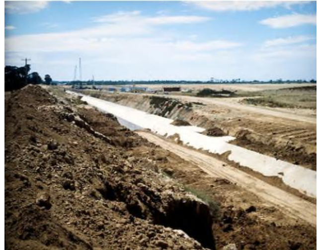
Figure 2-12: Construction of the WTS at Farm Road on 25 July 1983 (Melbourne Water)
