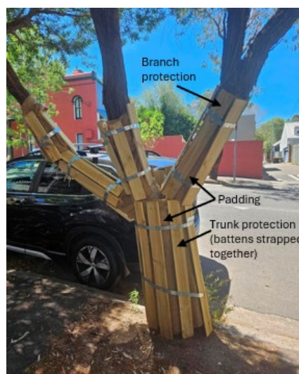
Figure 8: Trunk and branch protection
