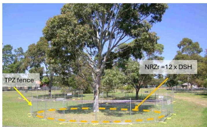
Figure 4: Tree protection fencing is erected around retained trees prior to site works
