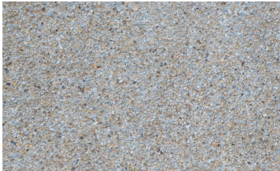
(A) Pavement - Lightly Exposed Aggregate In-Situ Concrete
