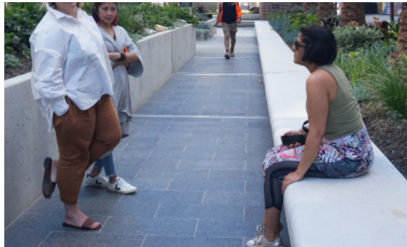
(B) Seating Walls - Precast Concrete
