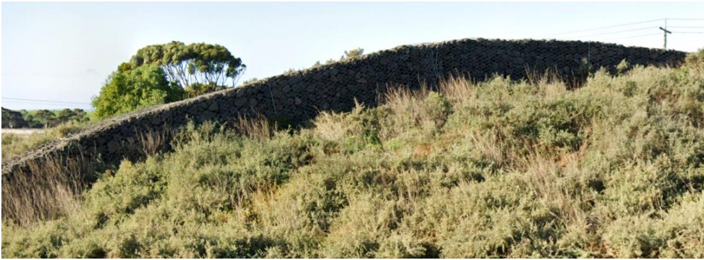
Figure 10 Gabion wall as curved landscape feature, M1 Highway / Geelong Ring Road, Victoria
