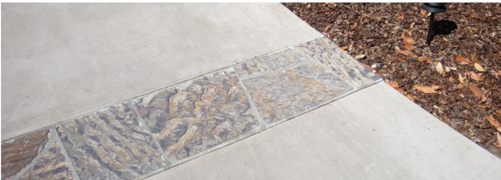
Figure 16 Stone inlay band in concrete
