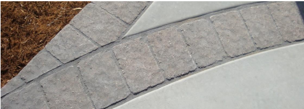
Figure 15 Paver band in poured concrete
