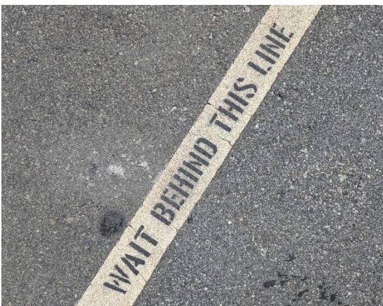
Figure 17 Examples of graphic markings applied on asphalt with road paint systems
