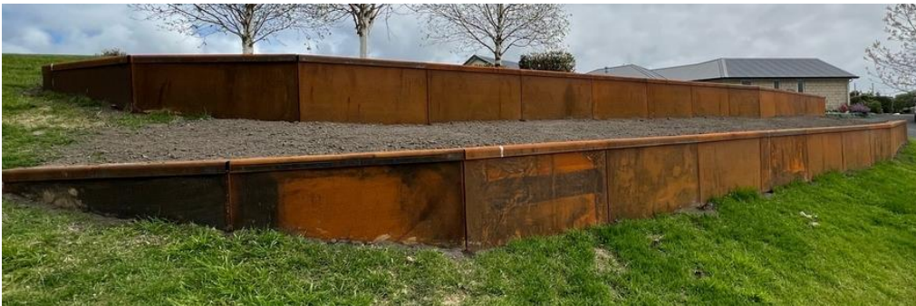
Figure 12 Corten retaining wall terracing, UK
