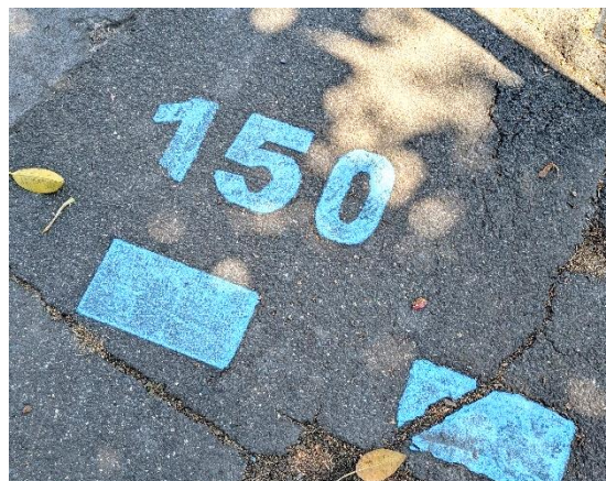
Figure 17 Examples of graphic markings applied on asphalt with road paint systems
