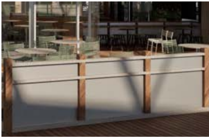
1 SGN-01 EXISTING BARRIER REFURBISHED - TIMBER AND NEW GALVENISED STEEL CLADDING
