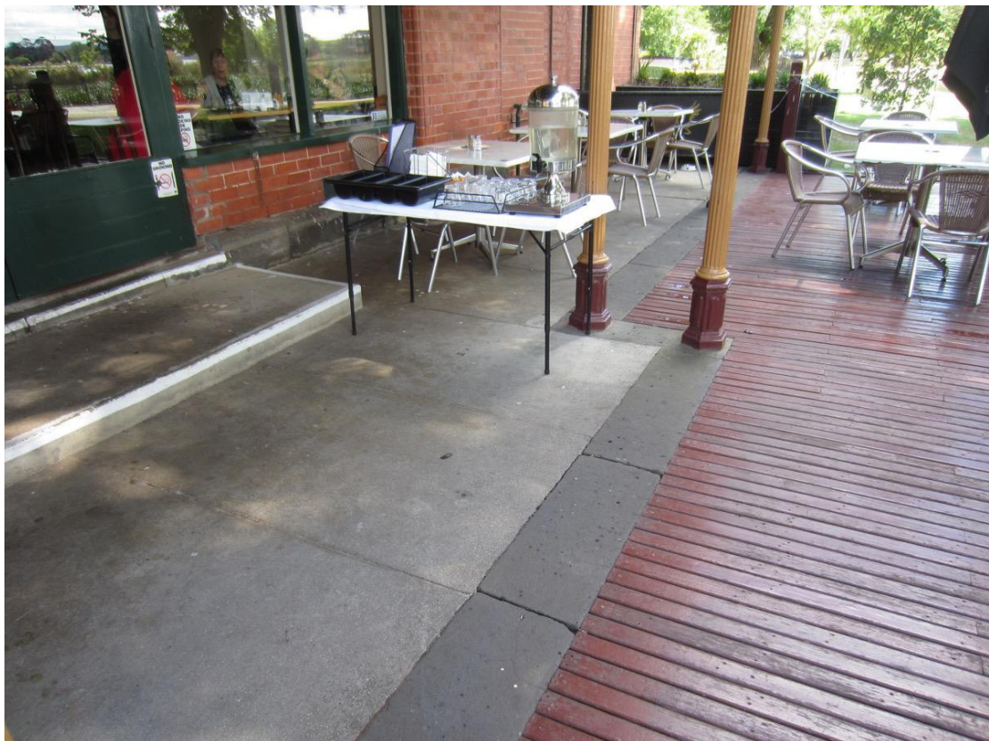
Figure 13 East verandah floor. The bluestone edging is original. The concrete surface has been altered with the step in front of the door added.
