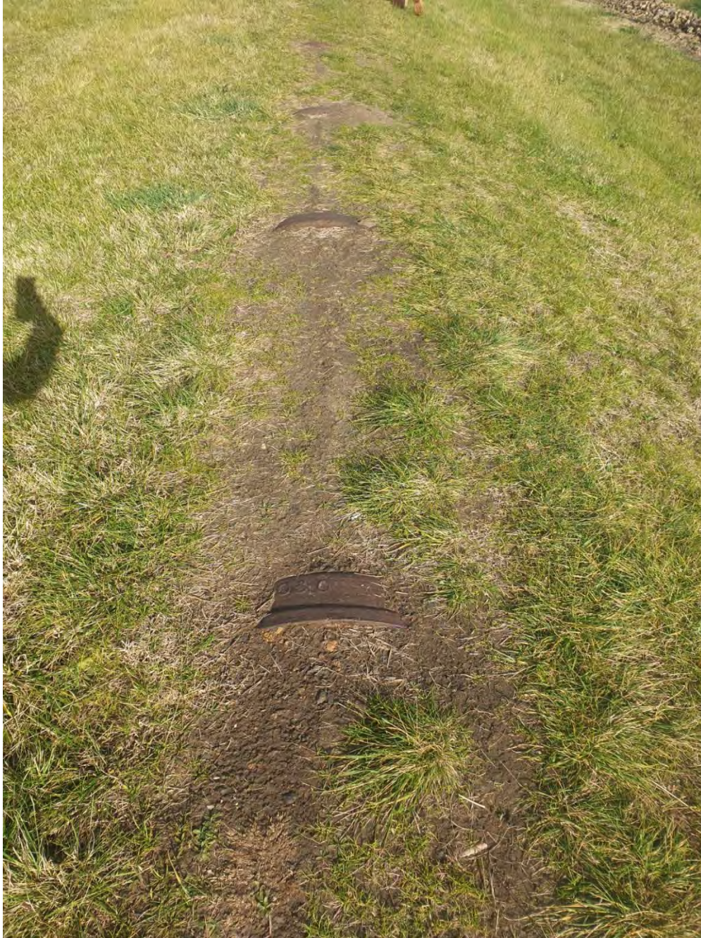
Figure 4.5 Exposed cast iron pipe joints at the northern extent of the study area. (Source: GML 2021)
