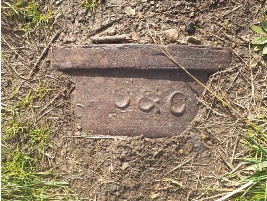
Figure 4.3 Exposed cast iron pipe with C & C embossing, northern extent of the study area. (Source: GML 2021)
