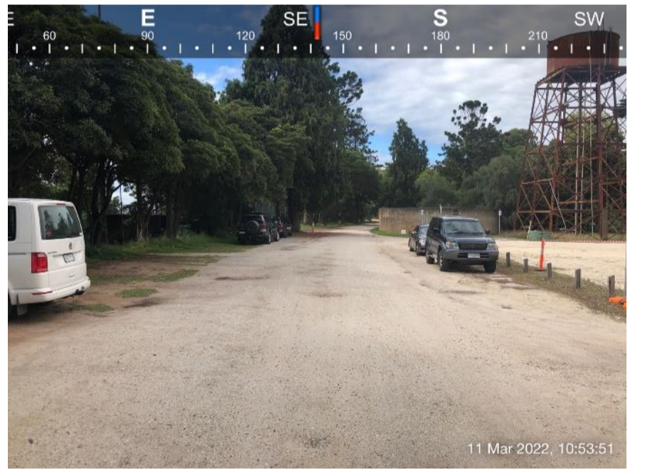
Figure 18: Southern Drive, a gravel roadway leading from Werribee Manion towards Shadowfax Winery. Location of proposed in-ground fire hydrant, inground sprinkler main, and in-ground dry fire conduit alignments
