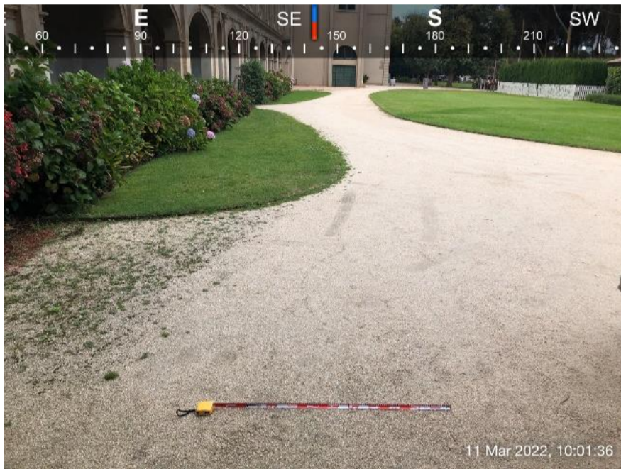
Figure 15: Gravel path and lawn surfaces between Werribee Mansion and mansion laundry. Location of proposed in-ground fire hydrant, inground sprinkler main, and in-ground dry fire conduit alignments
