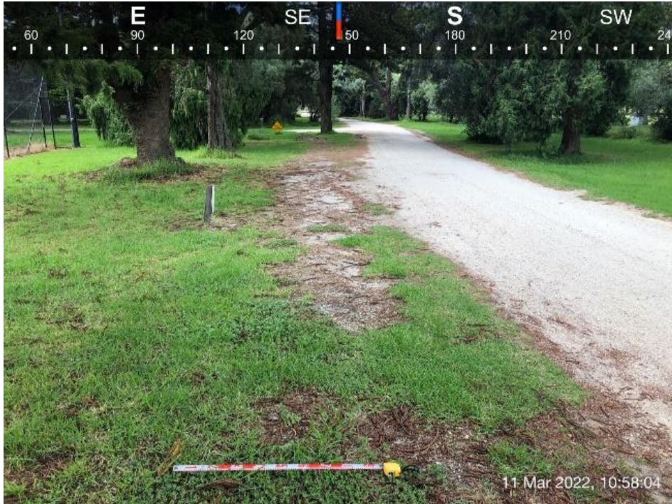
Figure 19: Southern Drive, a gravel roadway leading from Werribee Manion towards Shadowfax Winery. Location of proposed in-ground fire hydrant, inground sprinkler main, and in-ground dry fire conduit alignments
