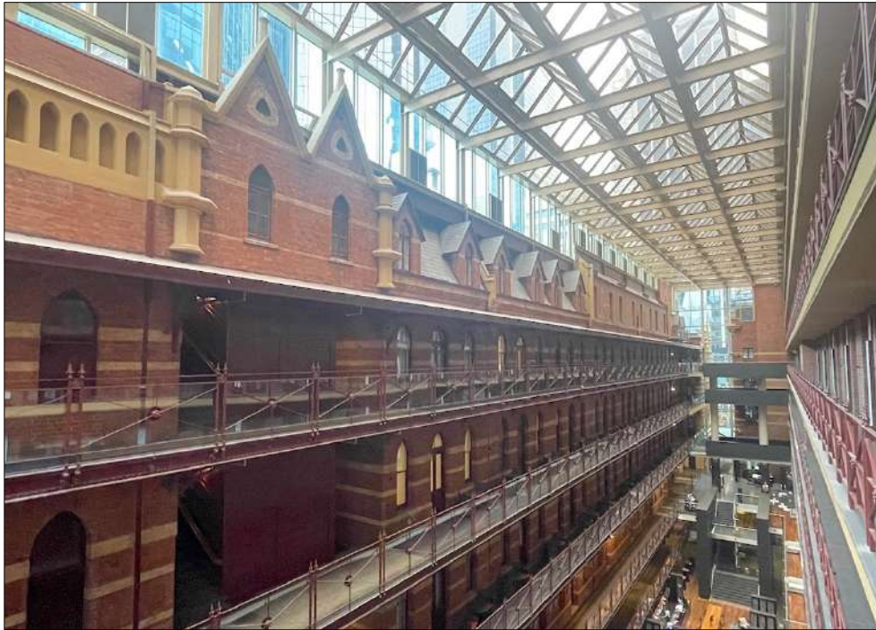
Figure 11 The east elevation and modern roof structure enclosing the hotel atrium.
