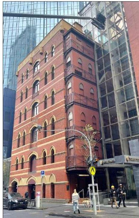
Figure 10 (right) The Flinders Lane façade with corrugated iron clad urinal enclosures.
