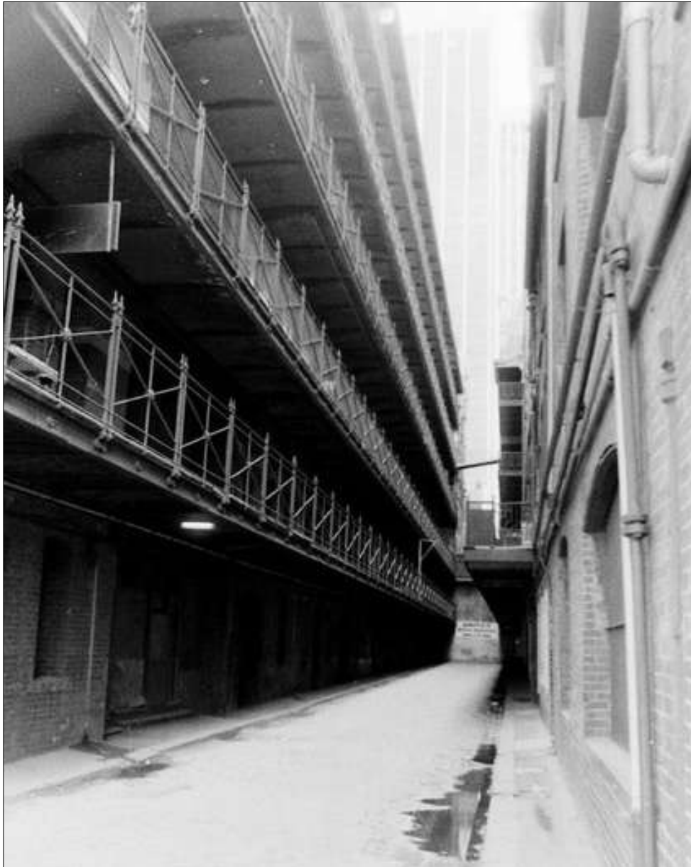
Figure 5 View from Winfield Square looking north, 1972. The Rialto Building is to the left. Source: Graeme Butler.
