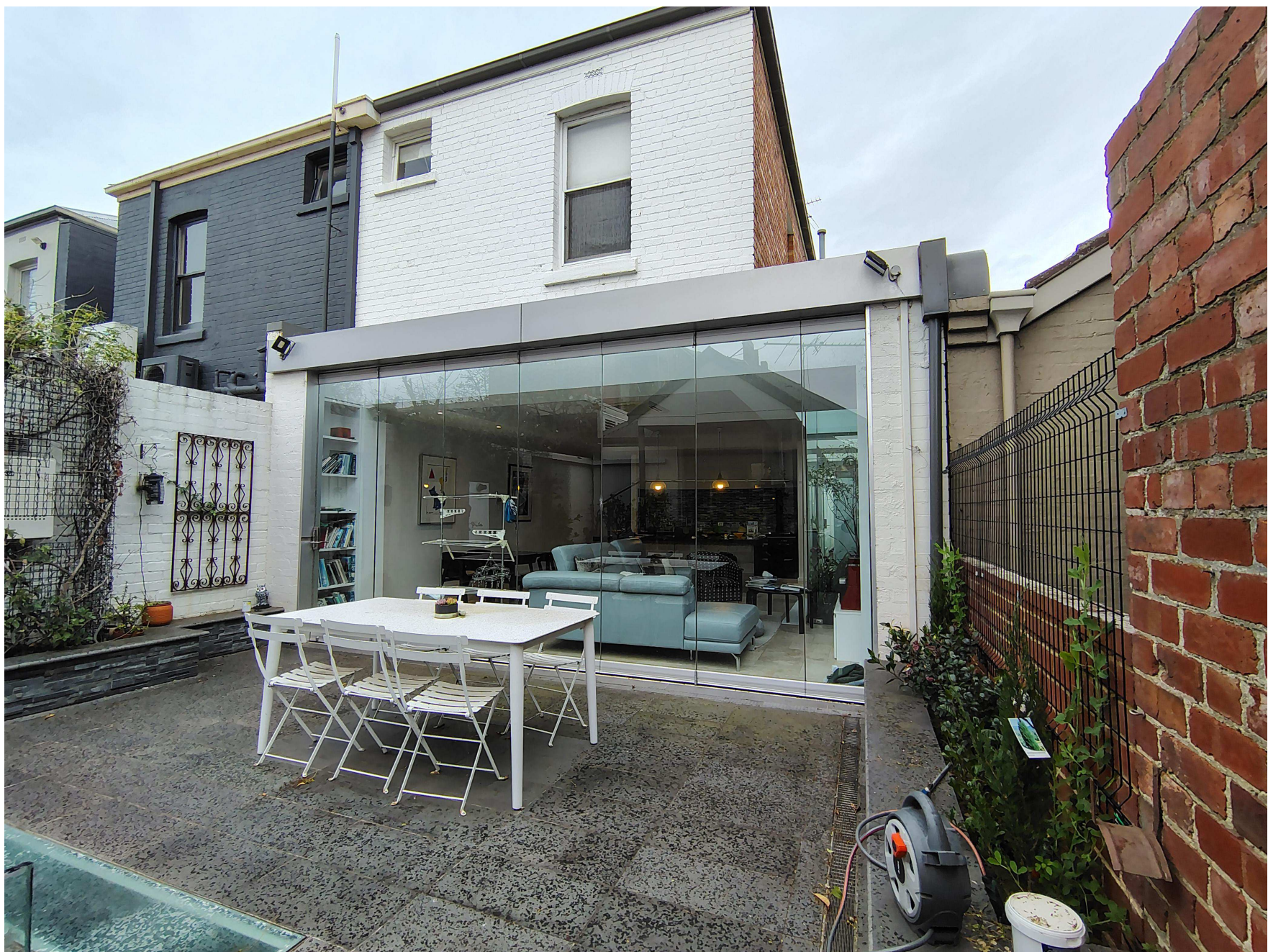
OBLIQUE VIEWSHOWING PAINTED BRICKWORK ON SUBJECT SITE AND ADJACENT
