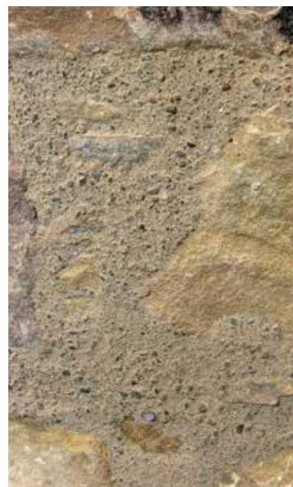
Figure 72: Tamped joints in rubble stonework. The tamped joints have a weathered or aged appearance with exposed sand grains. Without tamping, the colour would be that of the binder and finer sand grains. Also note the small pinning stones pushed into the mortar during repointing (see Chapter 22).
