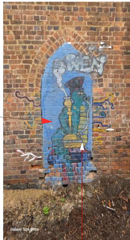
Location Of Toilet Block Opening Brick Infill To Be Remove
