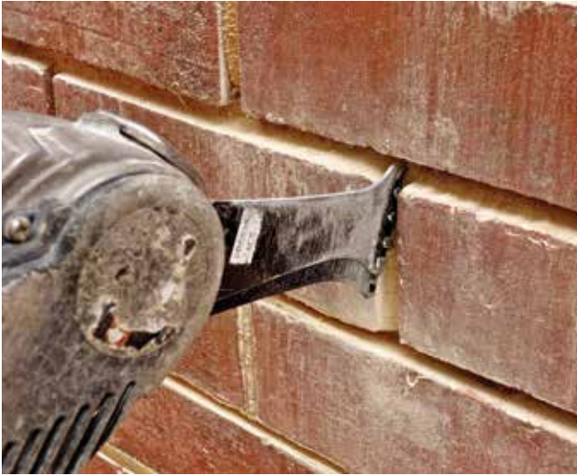
Figure 65: Oscillating-blade tools. These enable removal of moderately hard mortars while maintaining good control, reducing the risk of overruns. They are also much safer to use than rotating tools and produce less dust.
