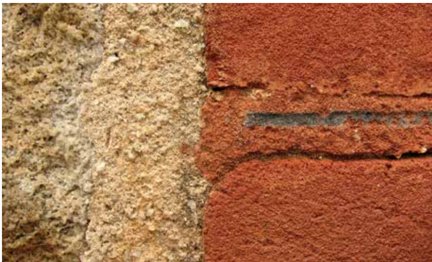
Figure 31: Pigmented mortar. The red pointing mortar, which matches the colour of the bricks, retains some of the black paint, termed pencilling, in the ruled joint. To the left, the white pointing tones-in with the sandstone on the far left.
