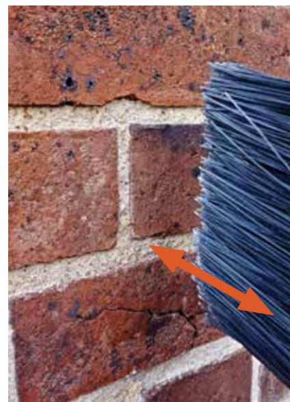
Figure 71: Tamping the joints. Tamping with a stiff-bristled brush (such as this churn brush) produces an aged appearance.
