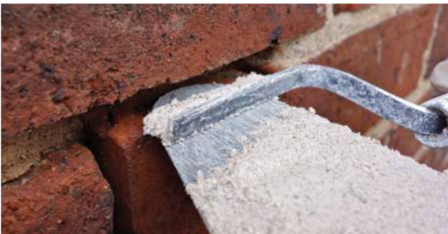
Figure 69: Using a trowel as a hawk. Speeding up delivery of mortar to a bed joint by using a gauging trowel as a hawk. Provided the underside of the trowel is kept clean, there need be no mortar stains on the face of the brickwork. A plastering trowel can be used in the same way.
