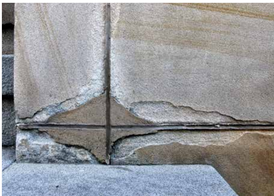
Figure 47: Inappropriate use of elastomeric sealant. Pointing the joints with an impermeable sealant has forced moisture to dry through the porous stones (rather than through the joints), resulting in salt attack decay to the sandstone. The damaged stones have been repaired with an equally impermeable patching material, forcing decay further through the sandstone.
