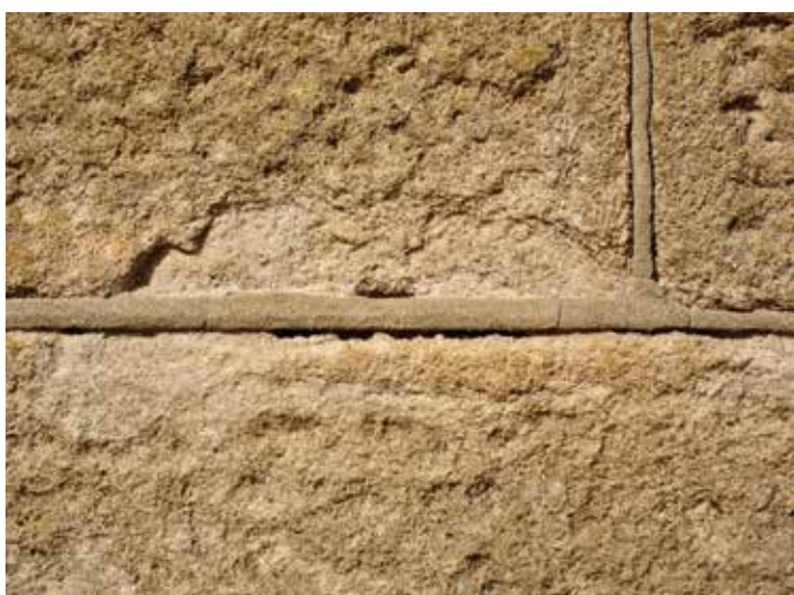
Figure 15: Impermeable mortar causing decay of adjacent stone.
