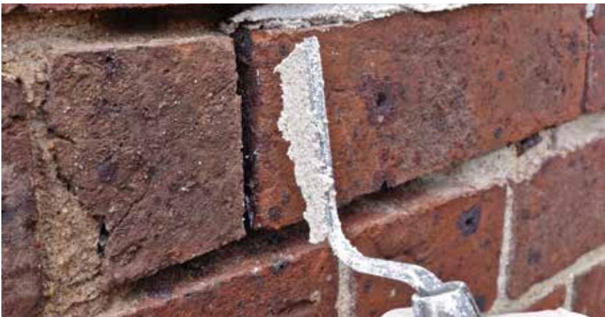
Figure 68: Filling a narrow perpend. Using a 4 mm wide trowel to place a thin wedge of mortar into a narrow joint. Careful placement with this technique removes the need to mask the face of the bricks with adhesive tape.
