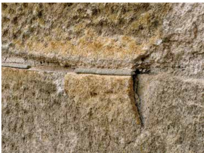
Figure 16: Spalling of edges due to thermal expansion.
