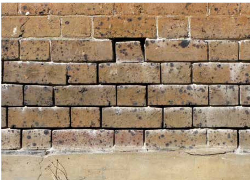
Figure 75: Mortar loss due to salt damp.
