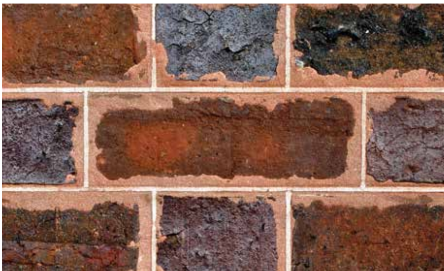
Figure 30: Tuck-pointed brickwork. The pale-red stopping mortar has faded from an original dark colour due to leaching out of the carbon black pigment. On completion, the stopping mortar would have been closer in tone to the surrounding bricks.
