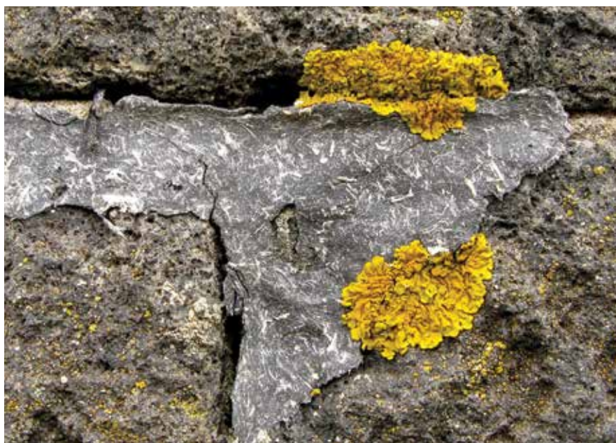
Figure 48: Old mastic sealant. The deteriorating sealant has pulled away from the adjacent stones, allowing water to enter the structure. Weathering of the sealant has exposed fibrous material which may be asbestos. Safety precautions must be taken when removing such materials (see Box 16 'Health and safety with mortars'). The bright yellow patches are lichens.
