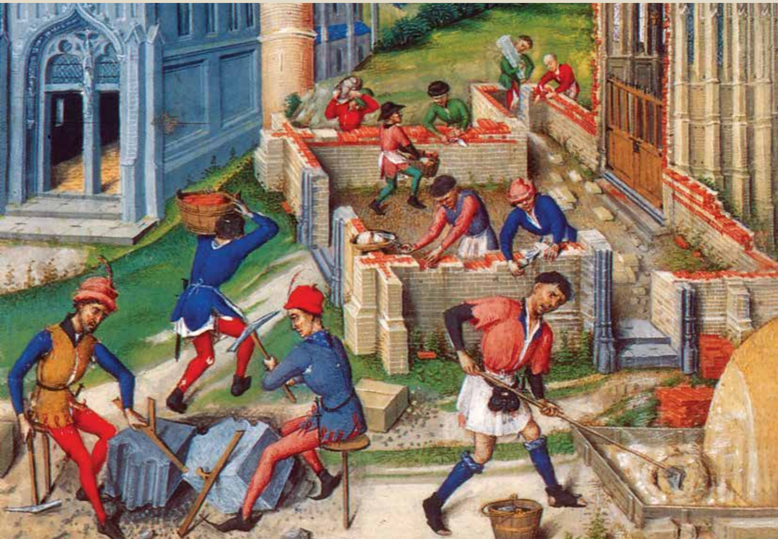
Figure 51: Medieval masons at work. Detail of an illuminated manuscript depicting the construction of a church in France, 1448. The labourer at the bottom right is knocking up some lime mortar with a larry (or mason's hoe), having cut it off as a slice from the maturing heap of banked mortar. This practice, including the kerbed, wooden platform (or stage) on which the mortar was mixed, was still in use in Australia in the late nineteenth century (see Section 15.1 'Traditional mixing'). Chronique de Girart de Roussillon . Codex 2549, folio 164, Austrian National Library, Vienna.
