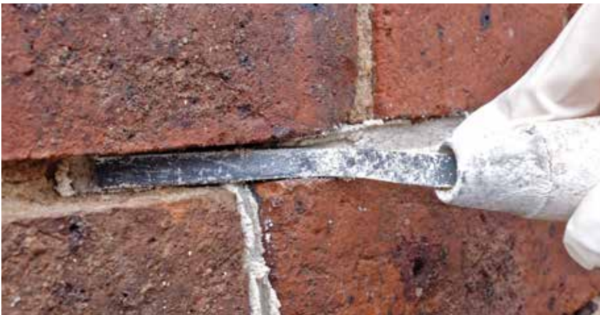
Figure 67: Filling a bed joint. An 8 mm trowel is used to place a small amount of mortar at the back of the raked-out joint; this is repeated until the joint is filled. The mortar is tightly compacted into the joint and also back into the last-filled section. This means working from right to left for a right-hander and left to right for a left-hander.
