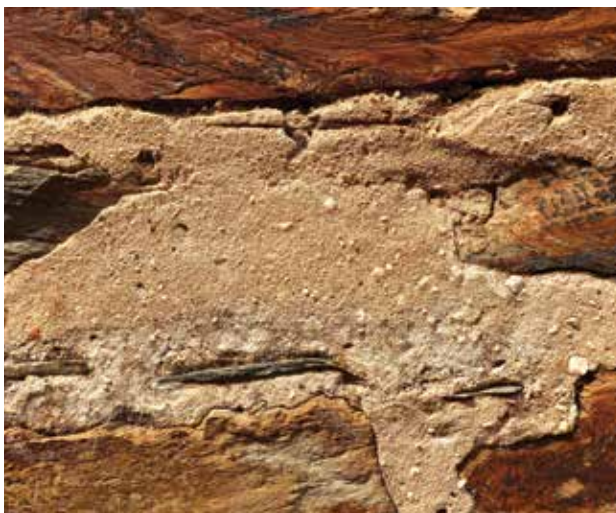
Figure 60: Flushed up pointing.
