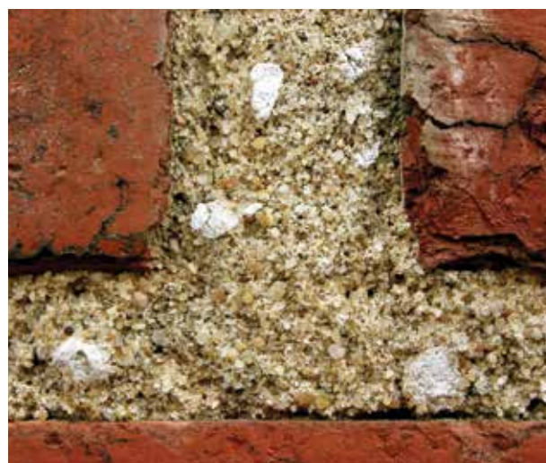
Figure 43: A 1920s mortar.
