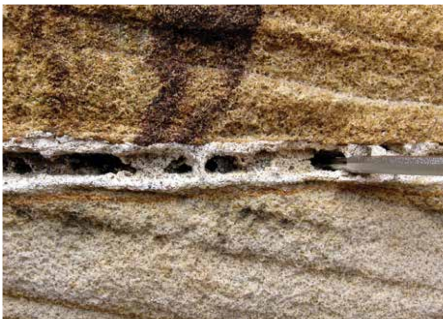
Figure 76: Mortar loss due to dissolution.
