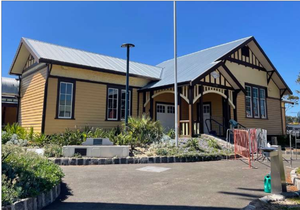
Figure 13 The west elevation of the main/upside platform building.
