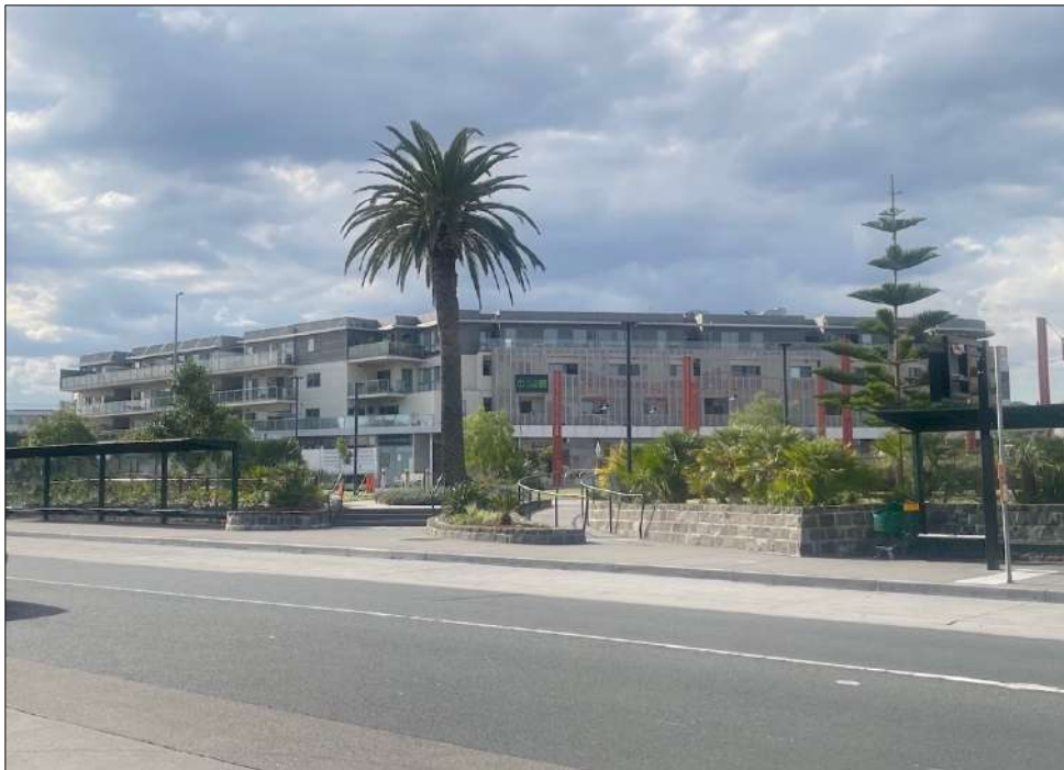
Figure 16 View north east towards the Mentone Railway Station gardens with modern four storey development in the background.
