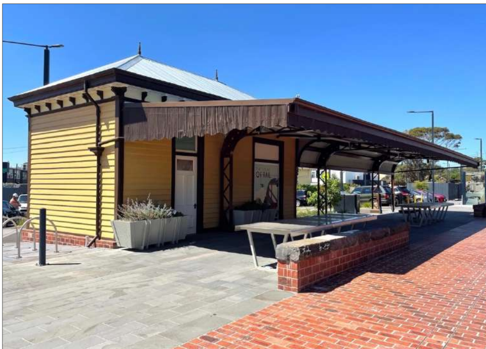
Figure 14 The downside platform building.
