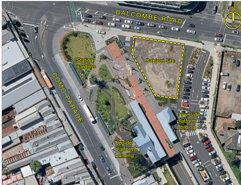
Figure 7 Aerial photograph of Mentone Railway Station and its environs.
