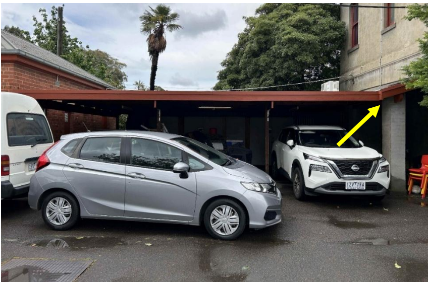
Figure 16 The existing carport and the verandah (as indicated) attached to the east elevation Source: Lovell Chen, 2025
