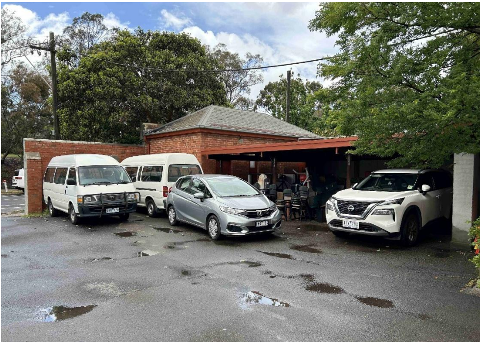
Figure 10 View to the carport adjoining the east elevation of Kawarau Source: Lovell Chen, 2025
