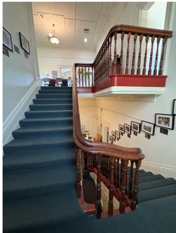
Figure 20 The main stair showing the existing original timber handrails and balustrades Source: Bryant Alsop, 2026
