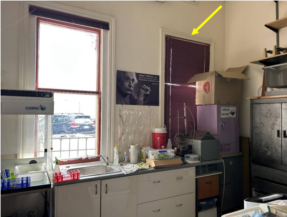
Figure 14 Existing window opening (as indicated) on ground level to be modified into a new door opening Source: Lovell Chen, 2025
