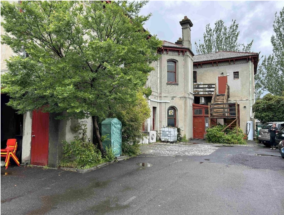
Figure 9 View along the north elevation of Kawarau Source: Lovell Chen, 2025
