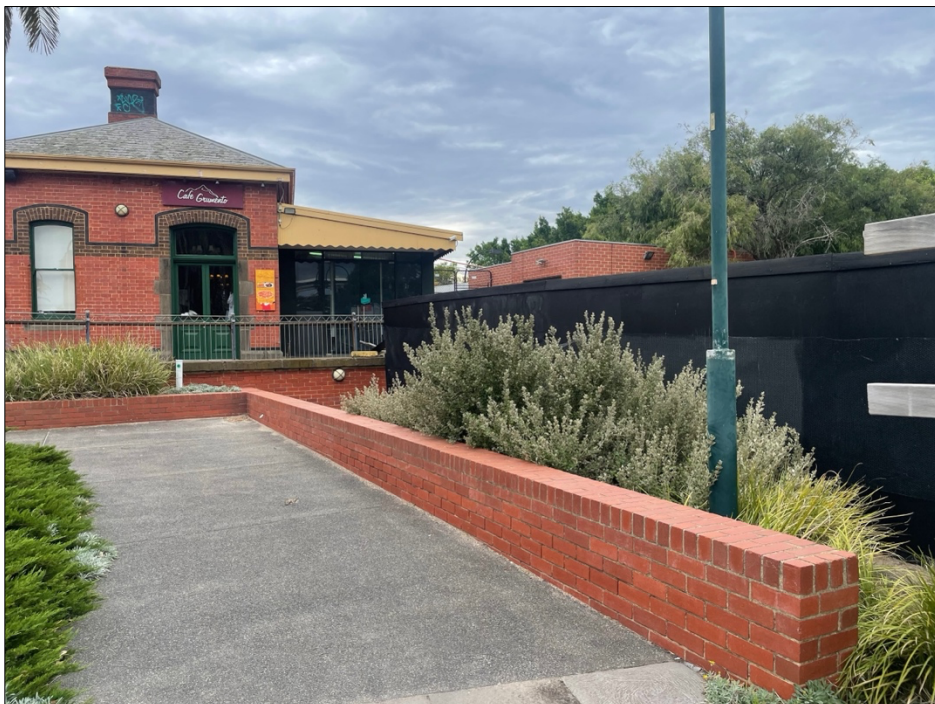
Figure 6 View of the red brick retaining wall/raised garden beds to the south of the station.
