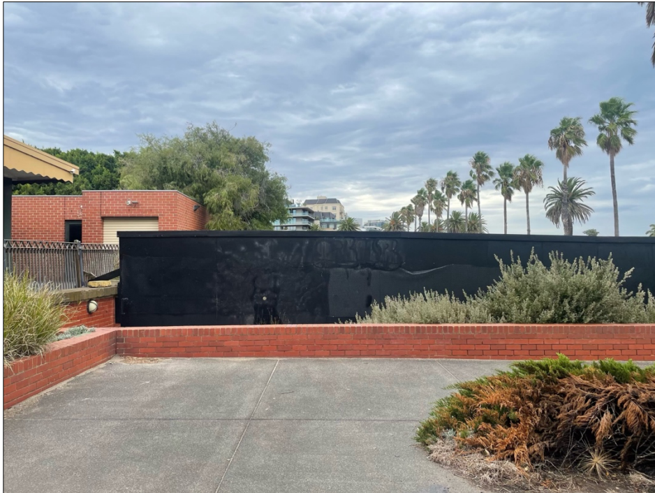
Figure 7 View east toward the subject site. The location of the tall hoard is approximately where landscaping works are proposed.
