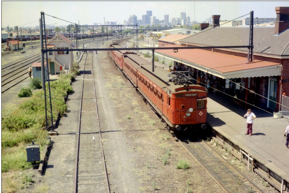
Figure 3 Oblique image of the Port Melbourne Railway Station c.1974. Image Source: Public Records office.
