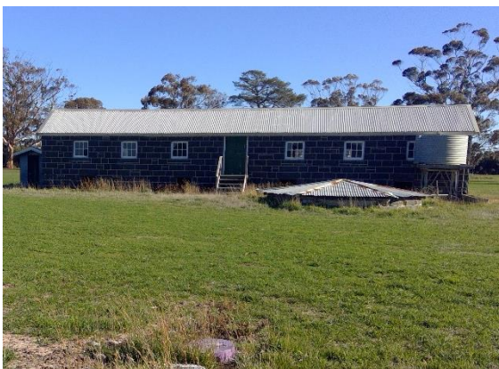
Figure 10: East Elevation of Rams' Shed with Cistern visible in foreground. Source: Trethowan Heritage, 2025.
