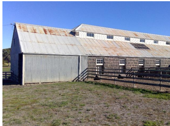
Figure 8: North elevation of the Woolshed. Source: Trethowan Heritage, 2025.
