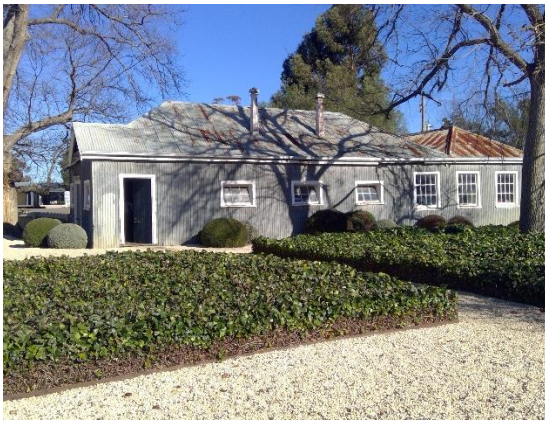
Figure 7: Engine house southwest of the Homestead. Source: Trethowan Heritage, 2025.
