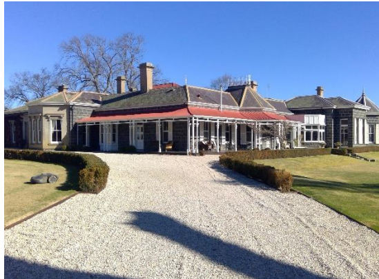
Figure 6: Northwest elevation of the Homestead. Source: Trethowan Heritage, 2025.
