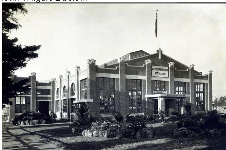
Figure 2, Woodfull Pavilion / Government Pavillion west facade (Melbourne Royal)
