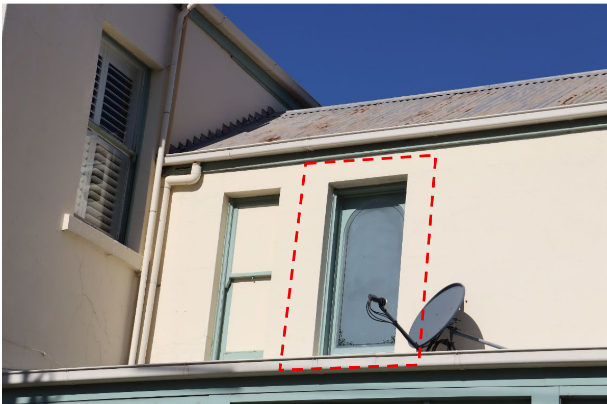
Figure 31. Original timber sash windows (one concealed internally) to rear of main wing and rear wing and non-original arched casement (dashed red).
