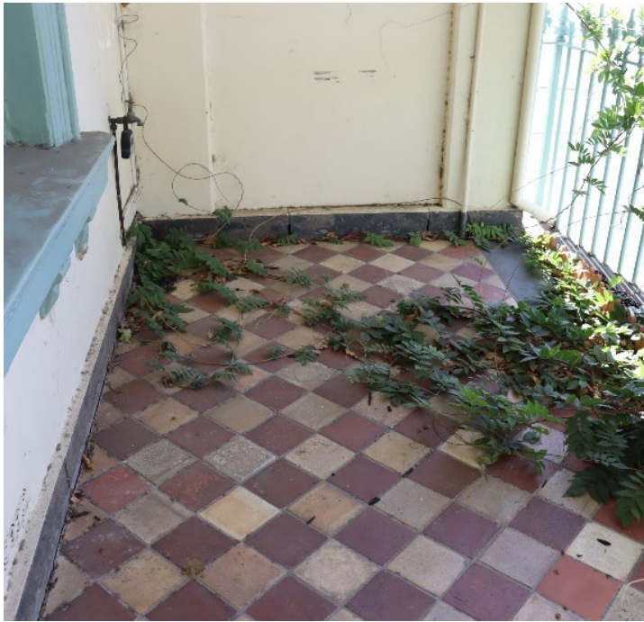
Figure 28. Verandah deck, tiles relaid, poorly.
