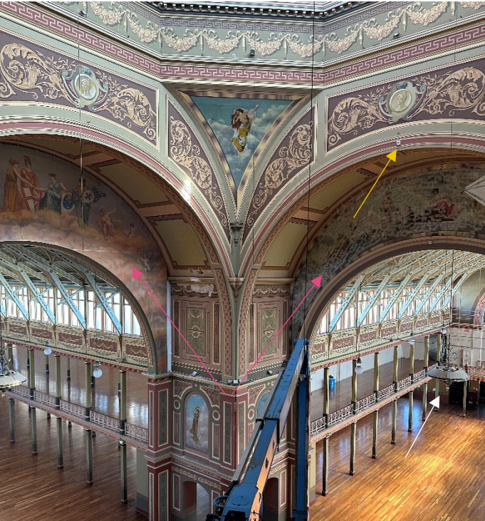
Figure 3 Lunette protection in the transept (pink), indicating location of vibration monitor (yellow) and gasolier (white).
