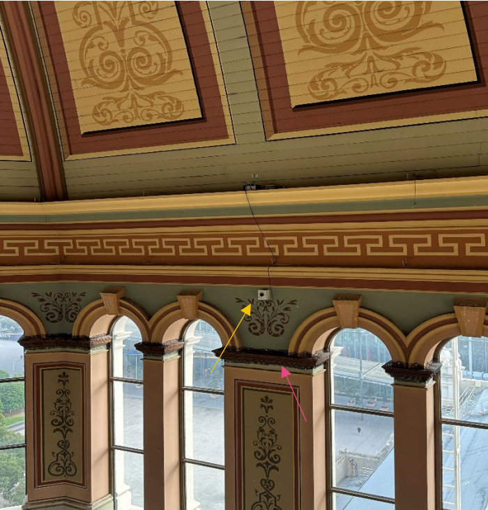
Figure 5 Netting of cornice in the dome (pink), indicating location of vibration monitor (yellow).
