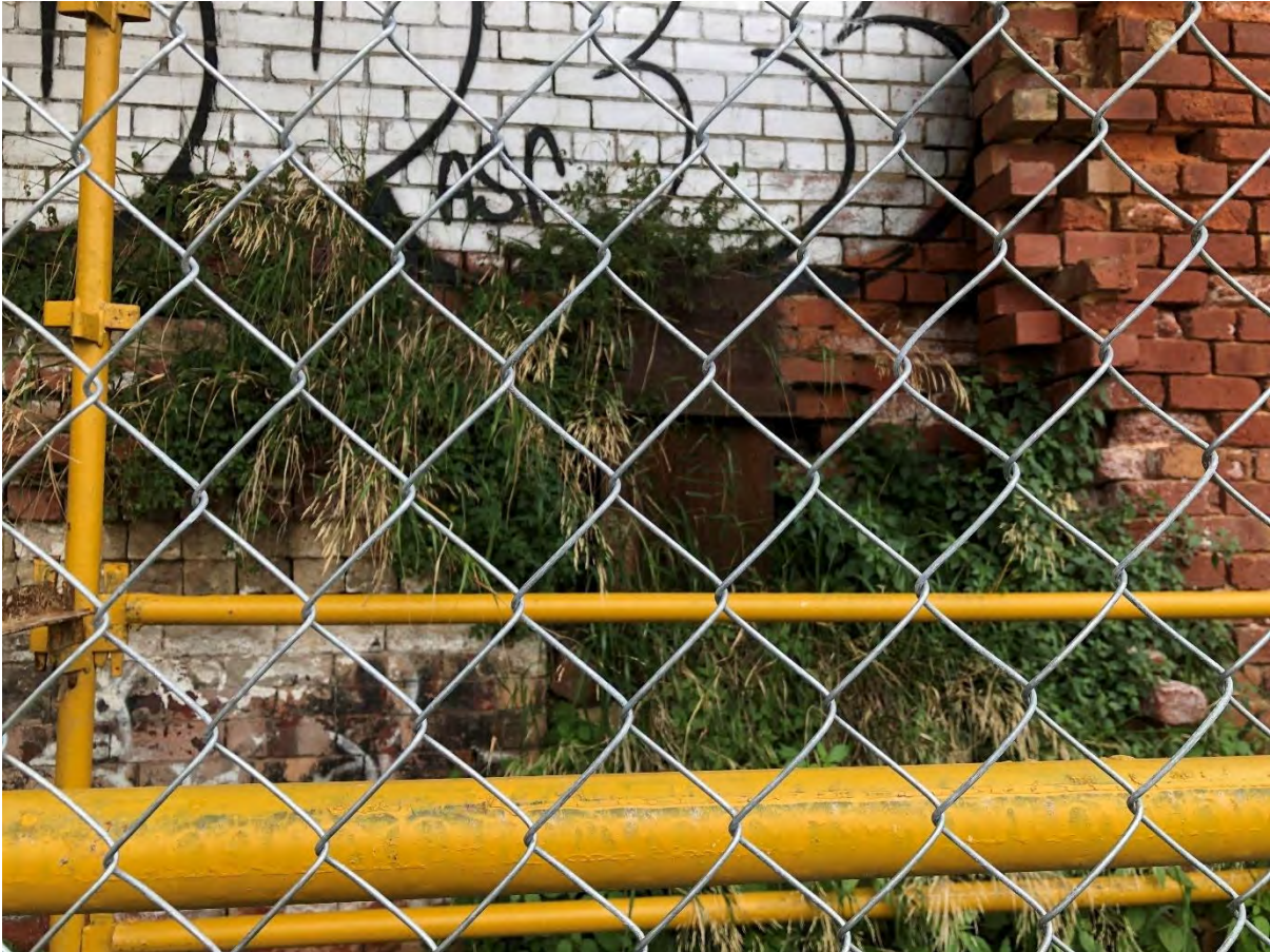
Image 5 – Existing Southern Wall
