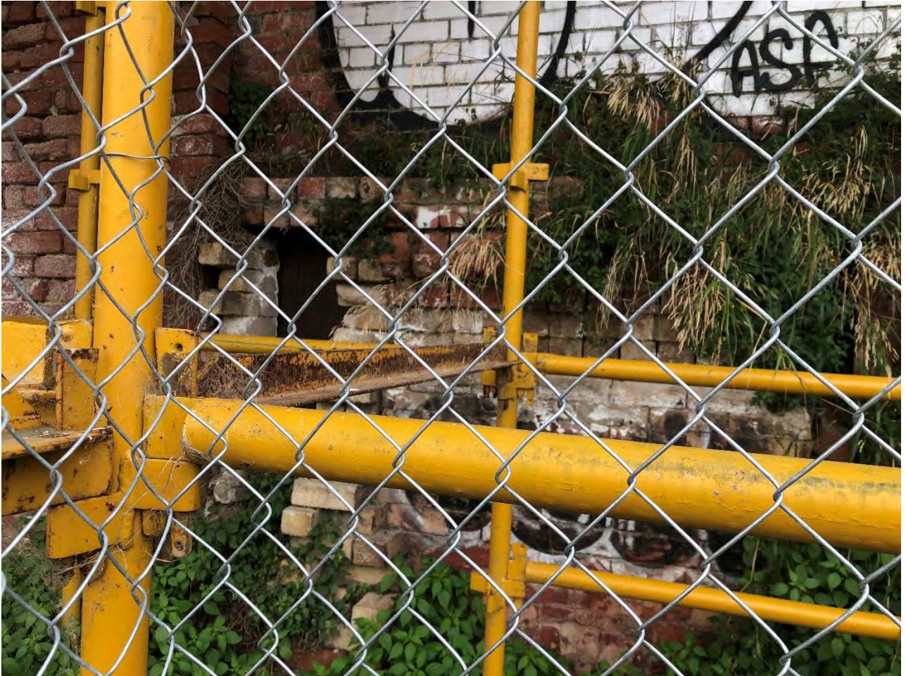
Image 4 – Existing Southern Wall opening
