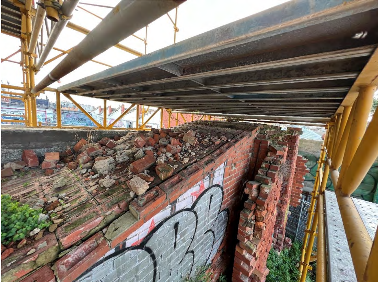
Image 15 – Existing Brick Roof
