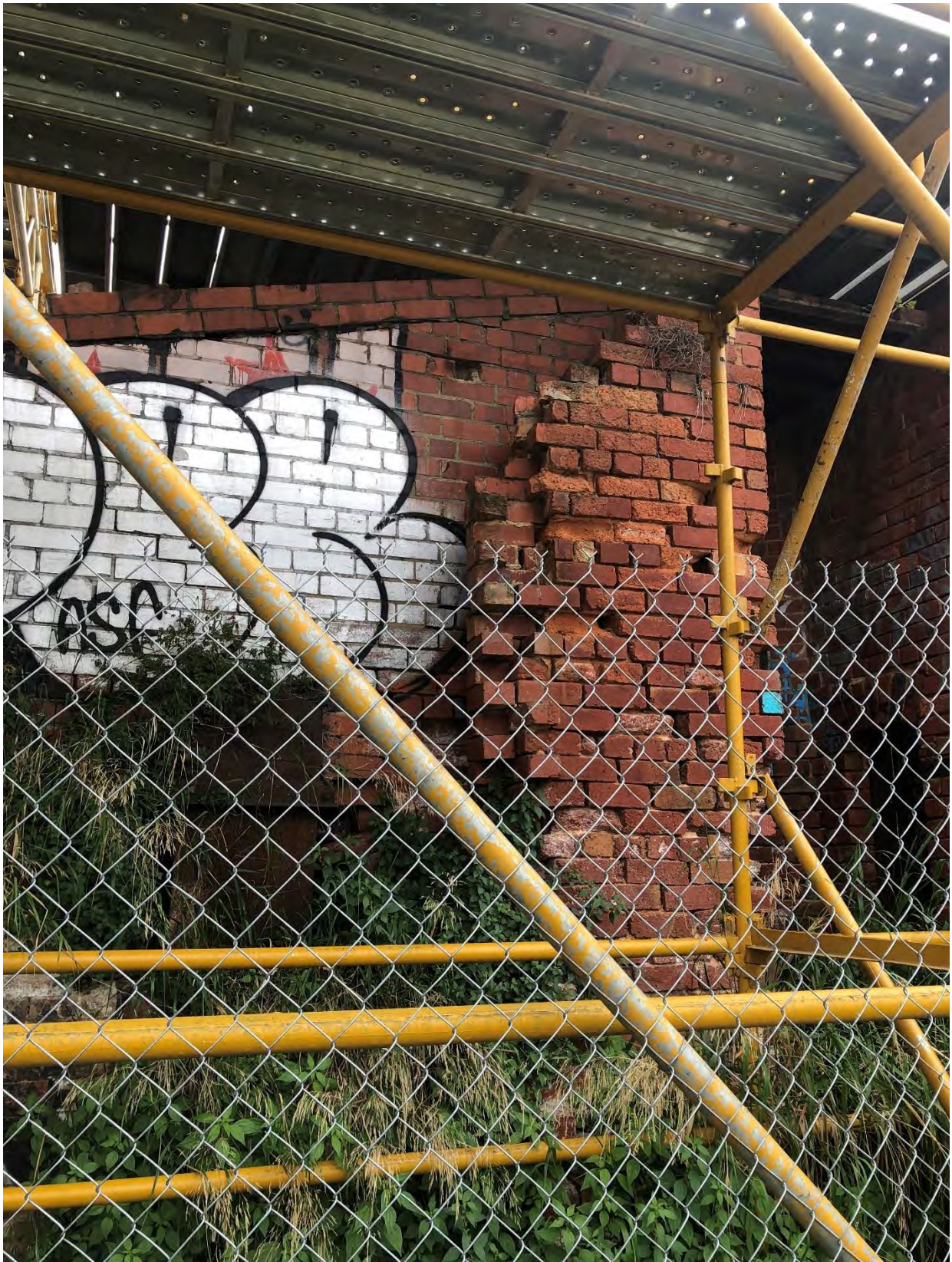
Image 3 – Existing Southern Wall
