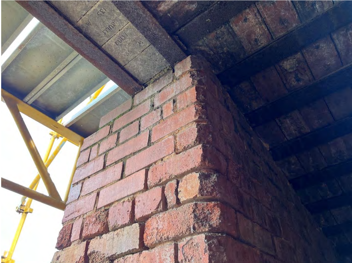
Image 21 – Existing Roof Soffit
