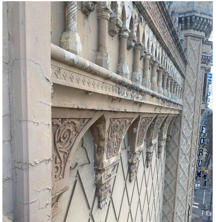
Figure 10 View of the cornice on the south elevation.
