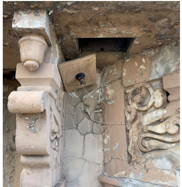
Figure 14 Corbels below tower balcony with suspended light fittings.
