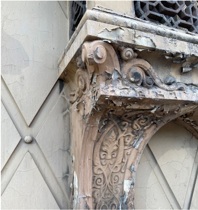
Figure 43 Cast cement groin vaulted brackets that support the balconies.
