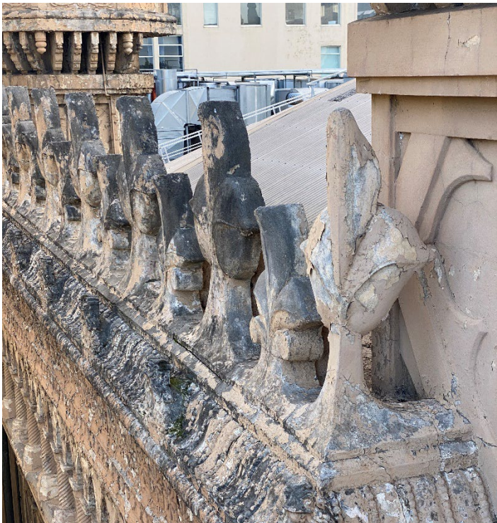
Figure 9 Typical details of the crenulated parapet.
