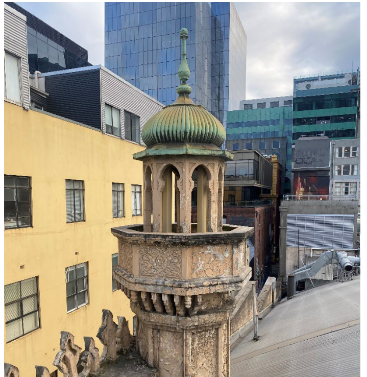
Figure 36 View of minaret on west elevation.
