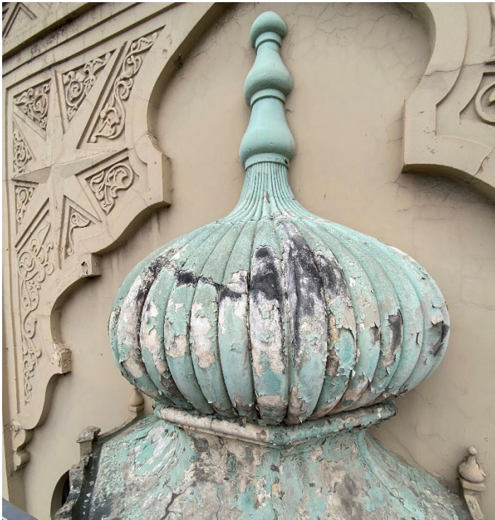
Figure 15 Canted bay balcony concrete dome roof.
