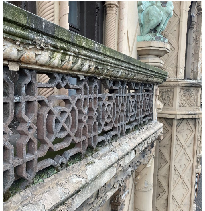
Figure 44 View of the balcony on the south elevation.
