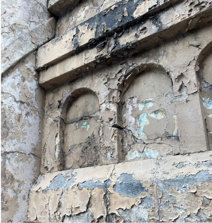
Figure 3 Crack in the concrete parapet on the east elevation – northern wing.
