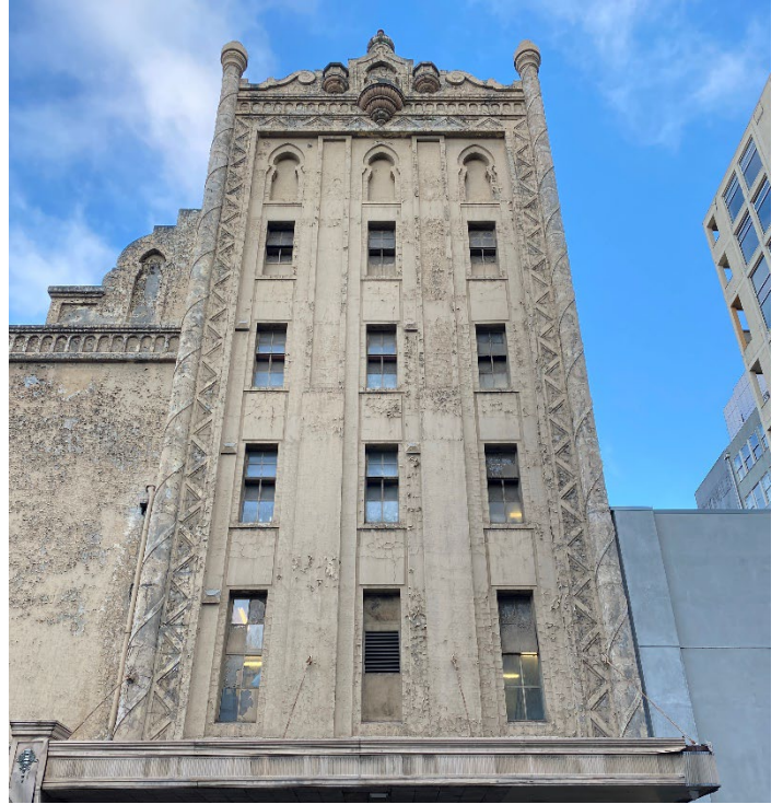
Figure 4 View of the northern wing on the east elevations.
