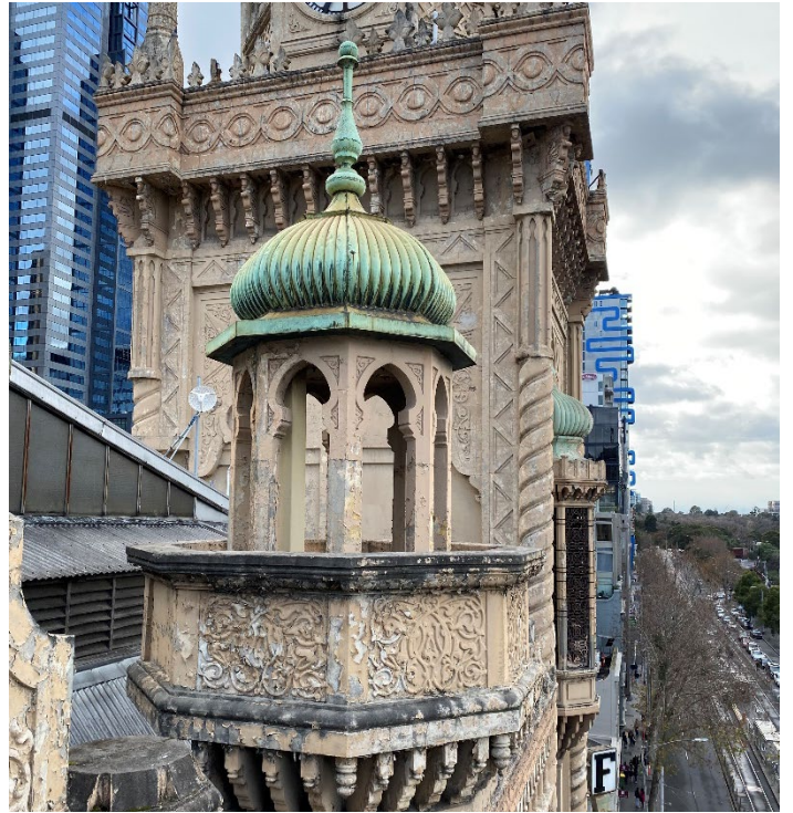
Figure 38 View of minaret on south elevation
