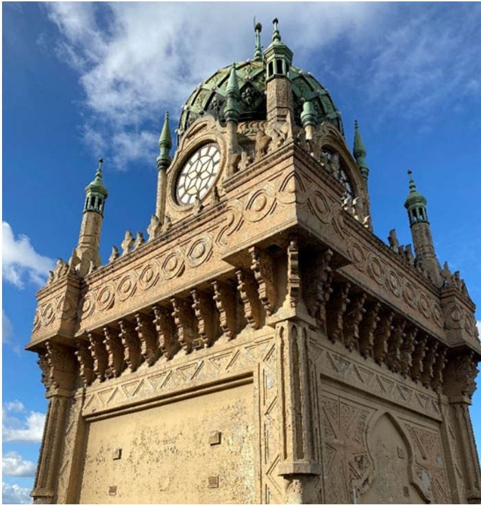
Figure 11 View of the tower from roof.
