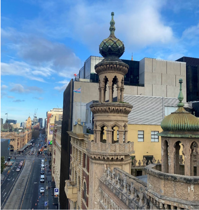
Figure 29 View of south west corner minaret.
