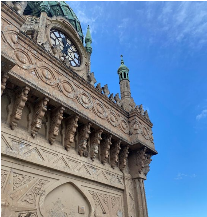
Figure 13 View of the tower balcony and upper walls.
