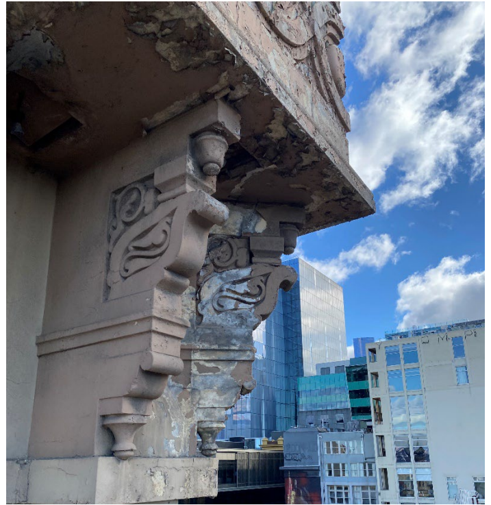
Figure 24 Detail of corbel brackets below tower balcony.
