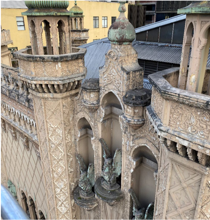
Figure 7 View of the south elevation parapet and niches.
