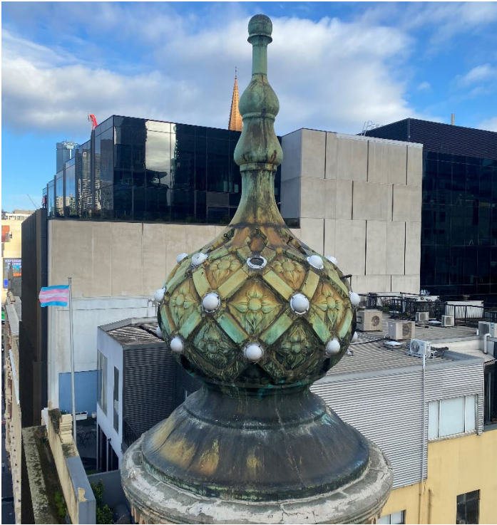
Figure 33 Onion dome over western minaret.
