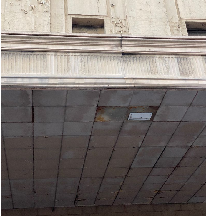
Figure 53 View of the canopy soffit showing the 1960s ceiling.
