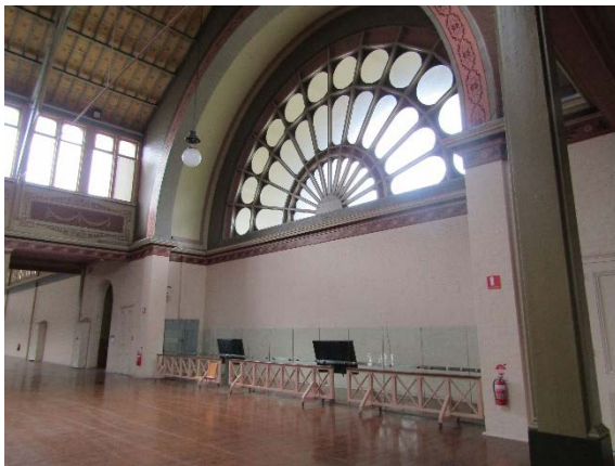
Figure 2.134 View toward southern gallery.
