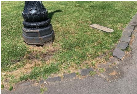
Figure 2.66 Eastern forecourt, proposed for VIP parking. Junctions of edging are vulnerable to damage at ends and corners.
