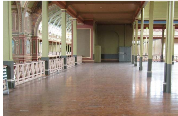
Figure 2.133 View in eastern gallery looking west.
