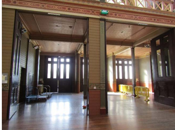
Figure 2.103 The timber fabric of the doors is potentially vulnerable to physical damage.
