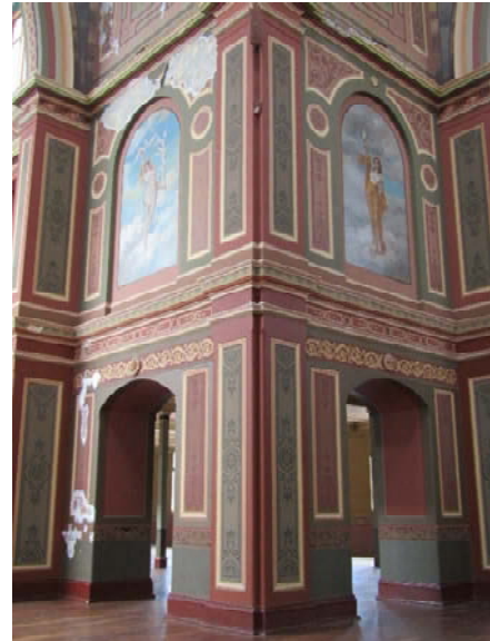
Figure 2.82 Detail of central pier in the centre of the Great Hall, showing partially completed conservation of decorative scheme.
