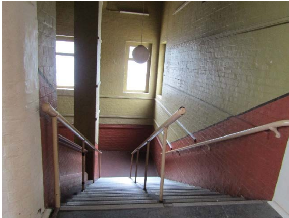
Figure 2.126 View of internal stairwell at the northern gallery.
