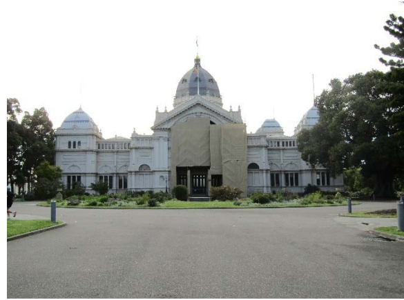
Figure 2.59 Western forecourt (looking east).
