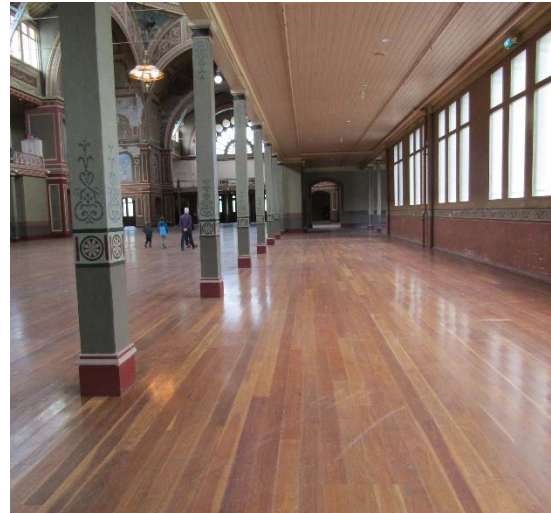
Figure 2.99 View from northern nave. The timber floor shows signs of general wear and scuffing.
