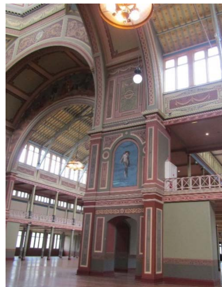
Figure 2.80 One of four central piers within the Great Hall.
