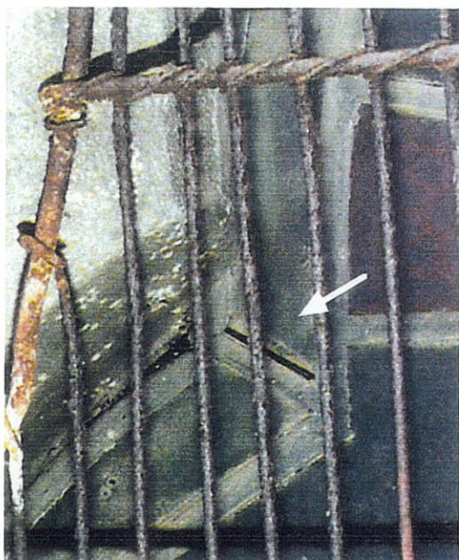
Exposed edges of glass, north nave
