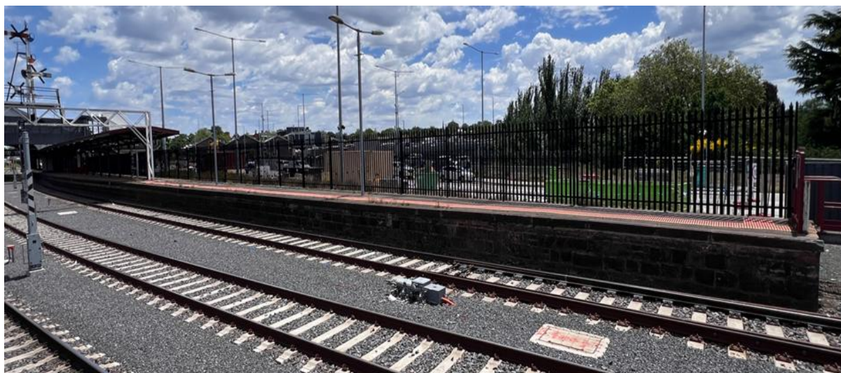
Fig.16. Platform 2 Up end to be rebuilt/realigned.
