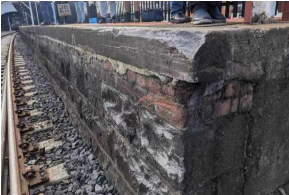
Fig.6. Up end of Platform 2 with strike scars.
