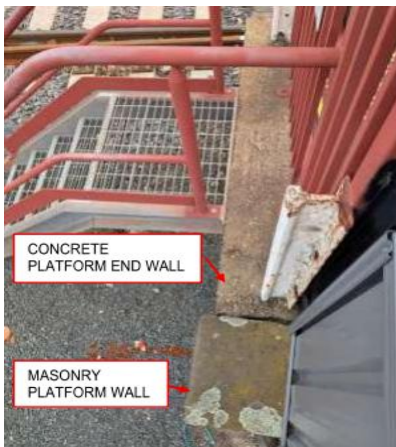
Fig.4. Up end of Platform 2 to be rebuilt.
