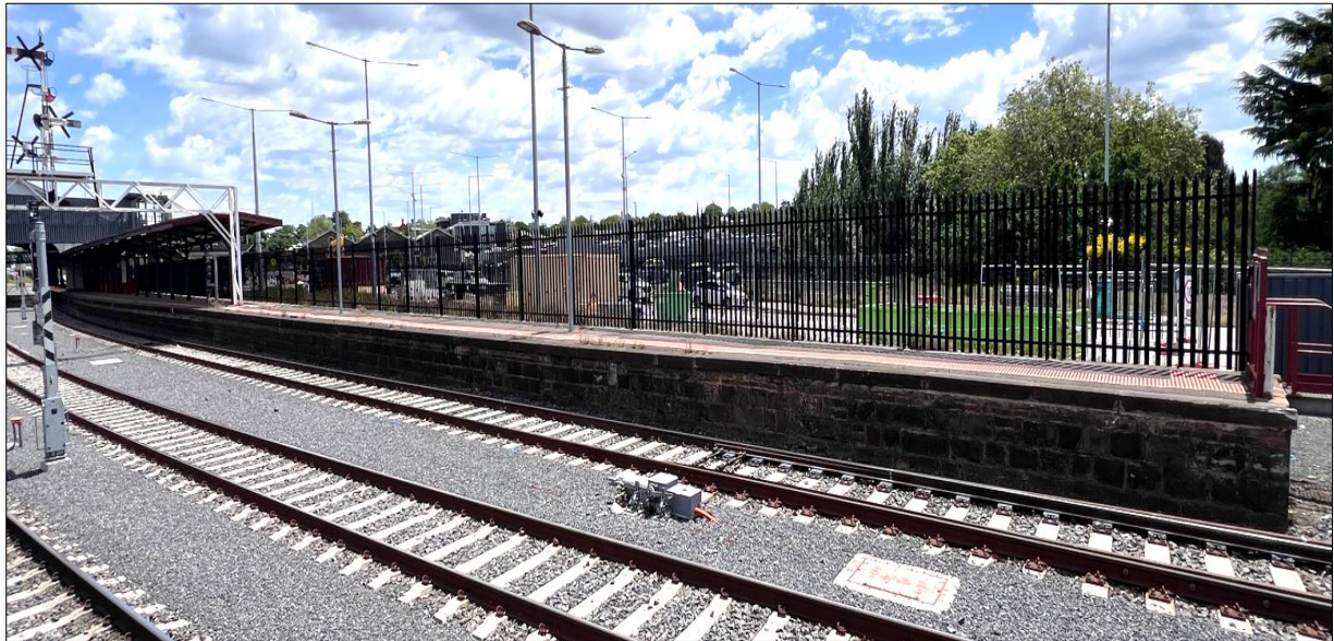
Up end Platform 2, Ballarat Railway Station 2025.
