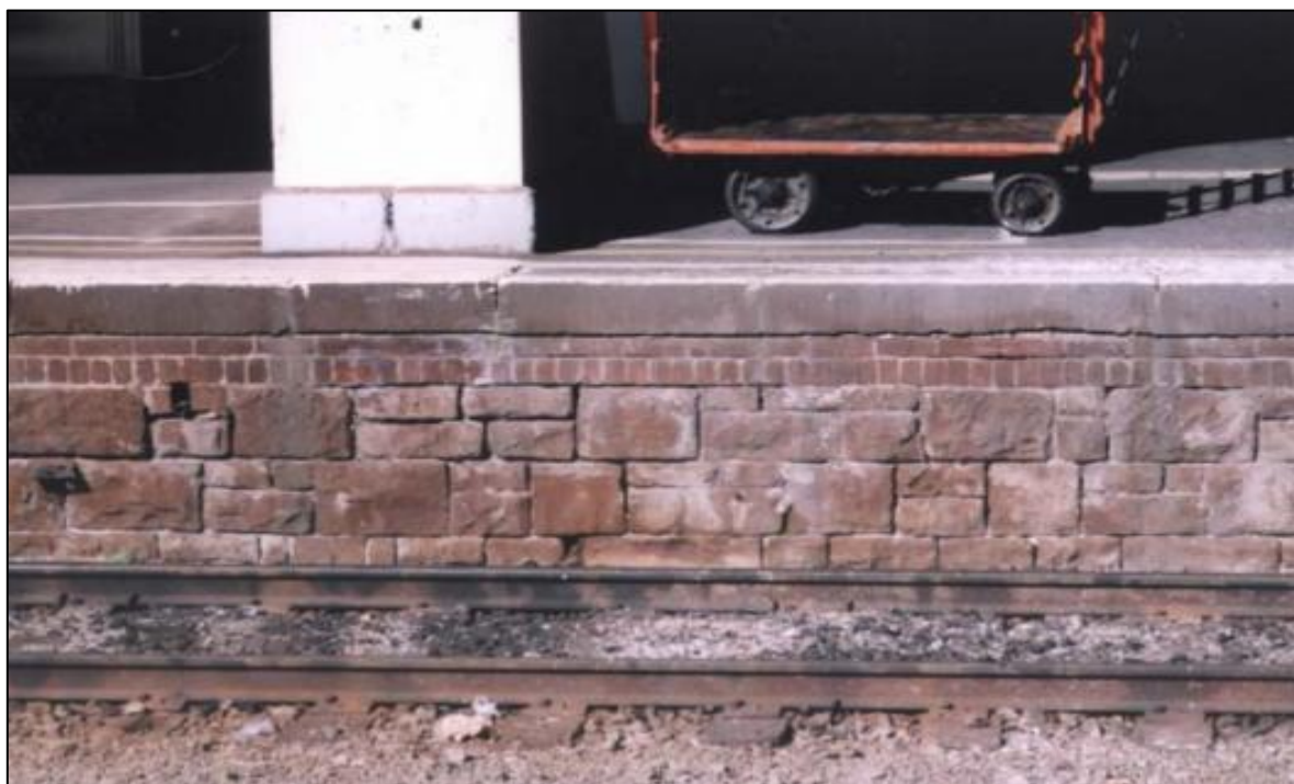
Fig. 17. The original station platform has been raised in height, as evidenced by the added courses of brickwork in the side walls visible in this image. (BRS CMP 2002:38).
