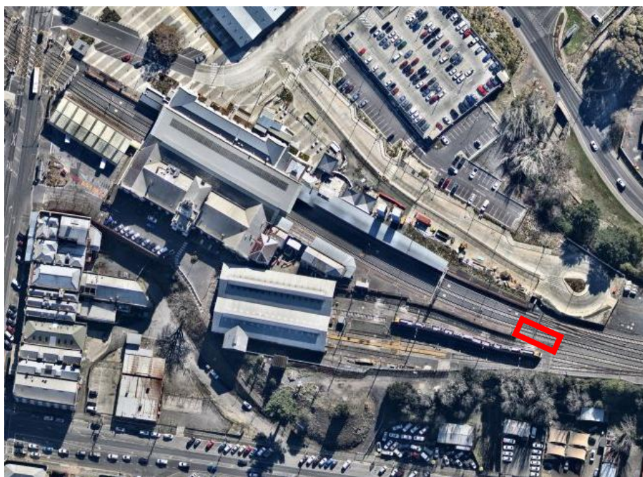
Fig.12. Works Area in reference to Ballarat Station
