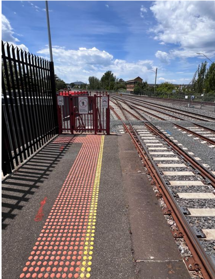
Up end Platform 2, Ballarat Railway Station 2025.
