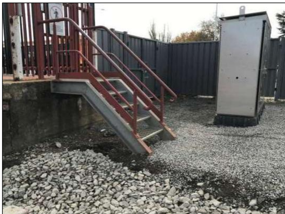
Fig.3. Up end of Platform 2 to be rebuilt.
