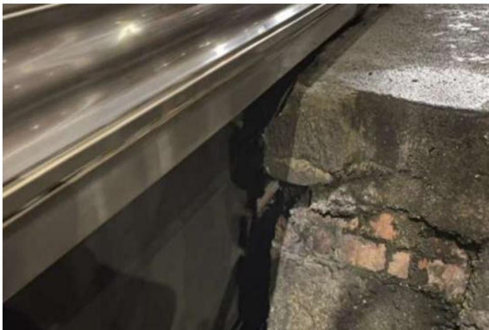
Fig.7. Up end of Platform 2 showing carriage interface.
