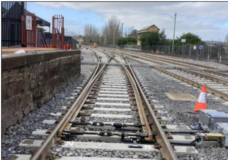
Fig.2. Up end of Platform 2 looking east.
