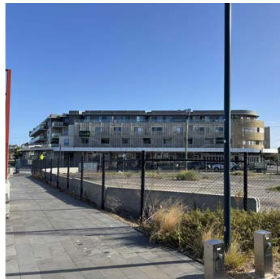
(B) 76 - 88 BALCOMBE RD
