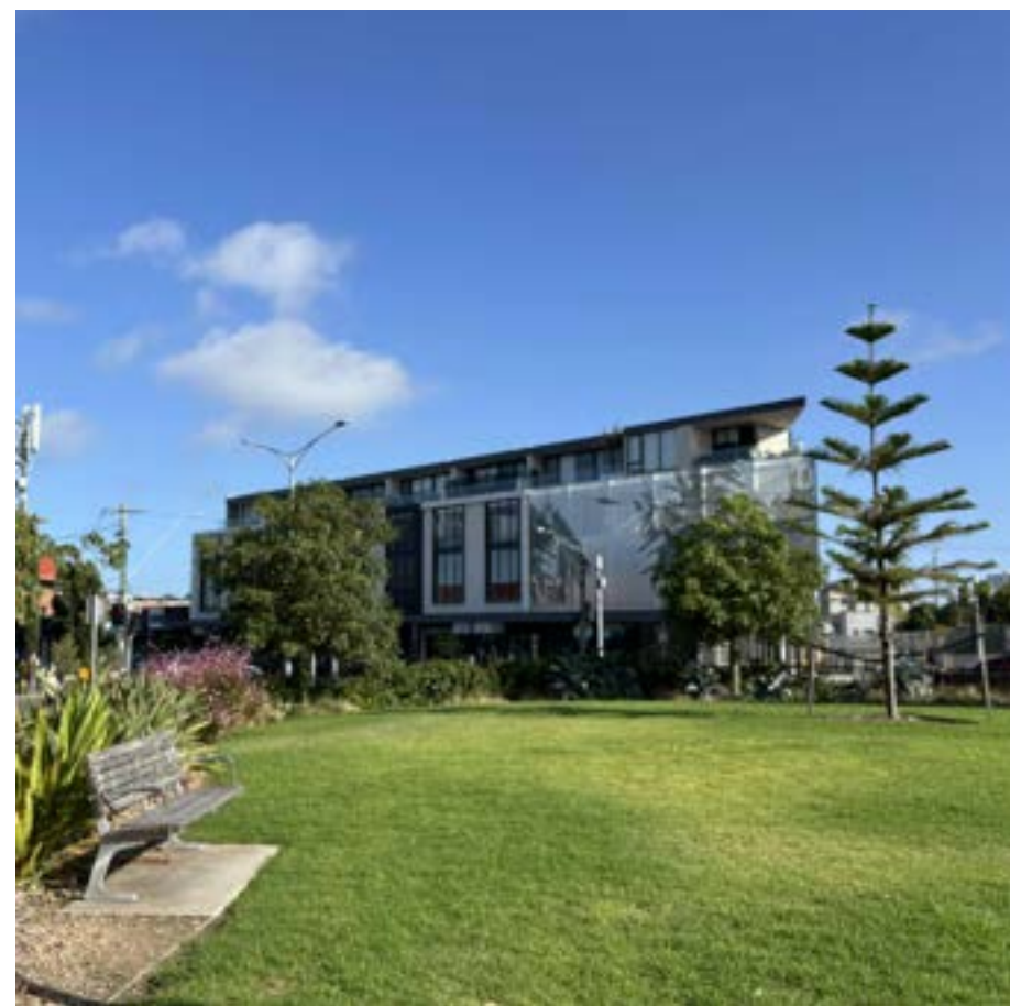
(A) 114 BALCOMBE RD
