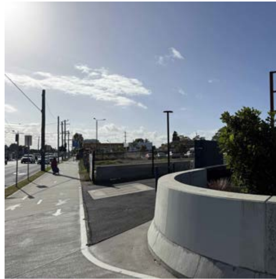
(C) VIEW EAST DOWN BALCOMBE RD
