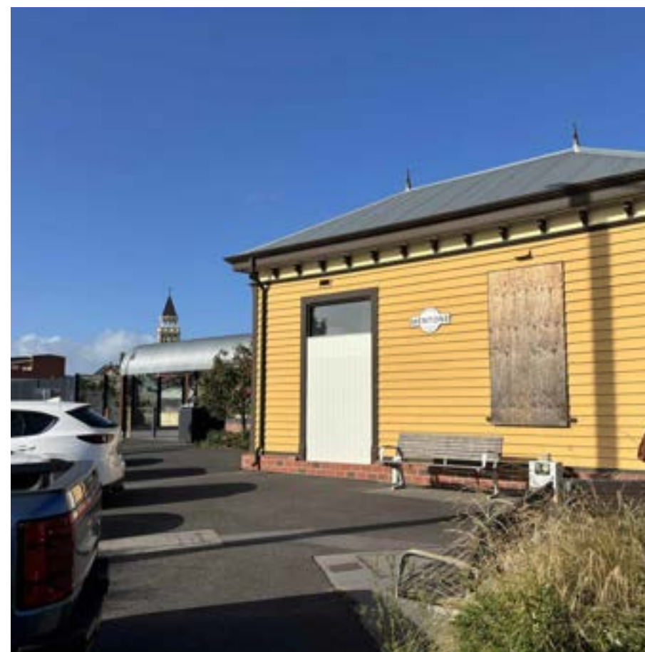
(F) REAR VIEW OF HERITAGE TIMBER STATION BUILDING
