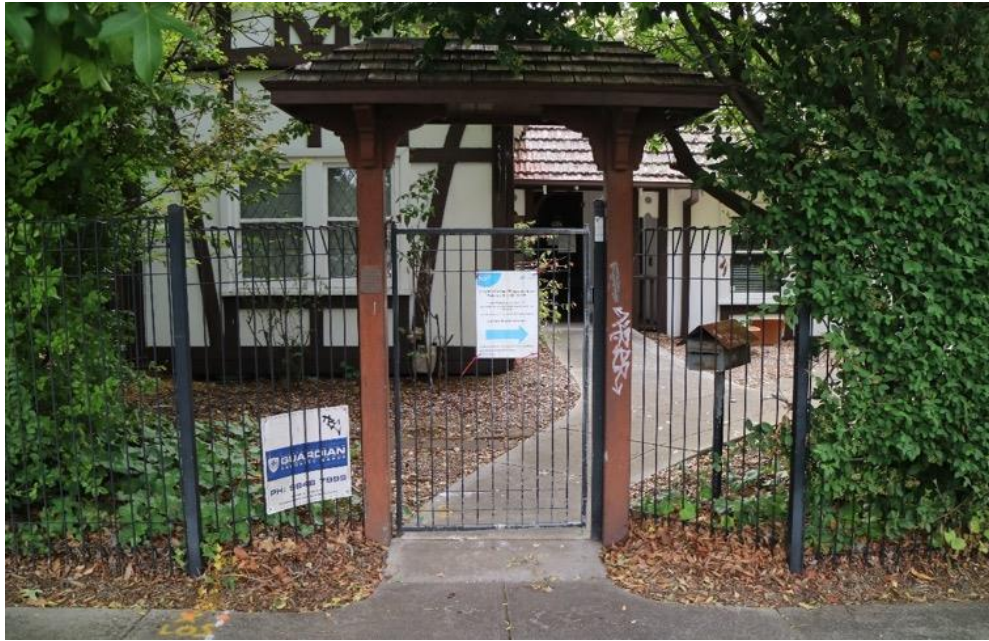
Figure 8. Closer view of lych gate (with later infill fencing) showing timber shingle roof and timber framing.
