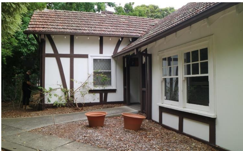
Figure 11. Looking north to main entry of building, showing imitation half-timbering, exposed eaves brackets, timber-framed sash windows, diamond pane glazing, etc.
