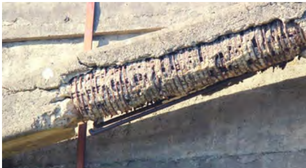
Figure 4 Example of reinforcement splice degradation (member ref 598)
