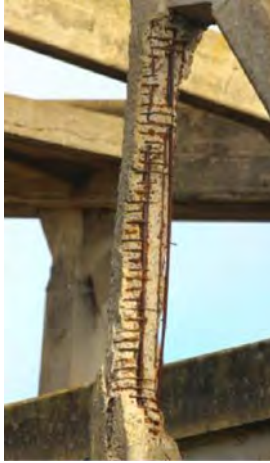
Figure 5 Example of main bar buckling (Member Ref 1032) – daylight visible between bar and core concrete
